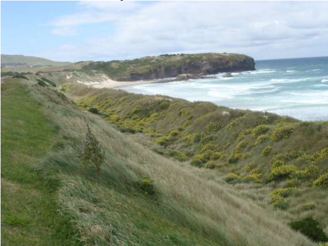
Figure 10 John Wilson Drive embankment showing the rear dune vegetation and embankment.
