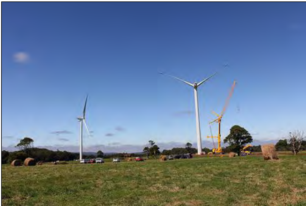
Hepburn Wind Farm during construction, 2011.
