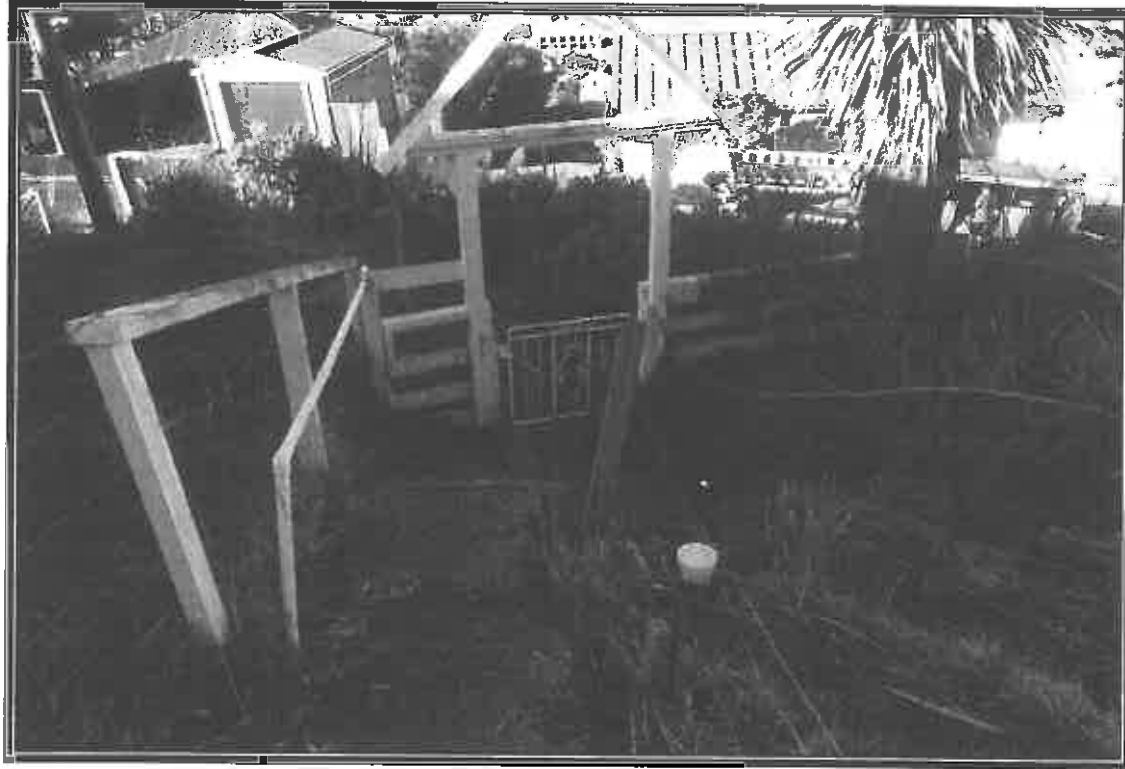
This photo shows the existing pedestrian access from the property to Cliffs Road through the archway shown in the photos above. The drainage cleaning eye is also in this view. (Taken August 2015)
