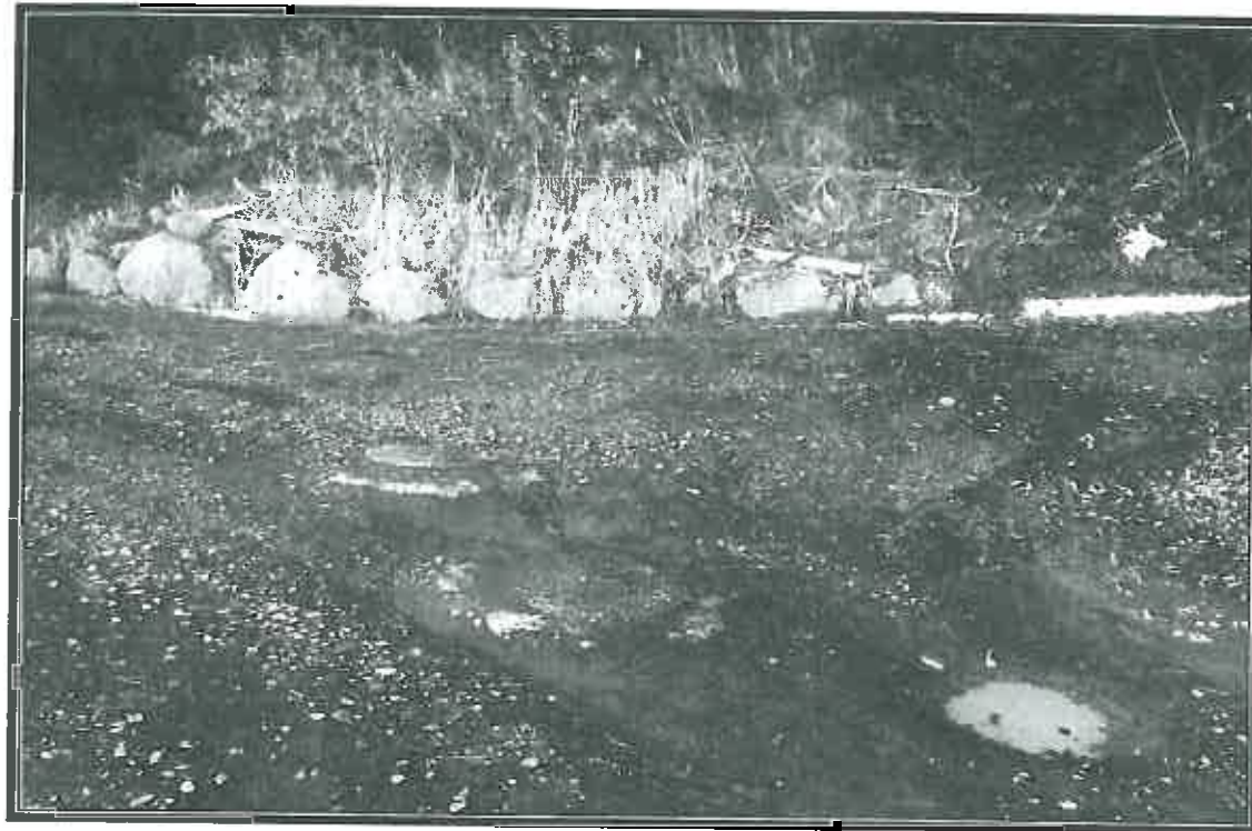
This photo shows the intersection of 'Lyders Road' and the driveway access to the subject site as well as the two manhole covers for the Stormwater and waste water sewers. (Taken August 2015)
