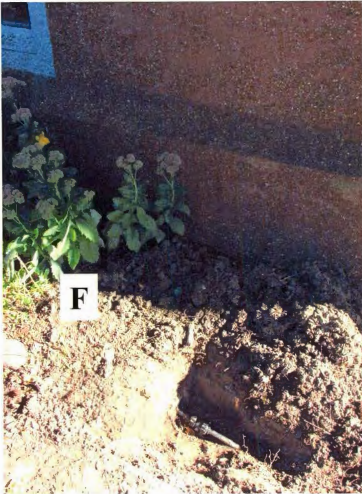
Figure 15 Repaired water pipe at location F (in Figure 7)
