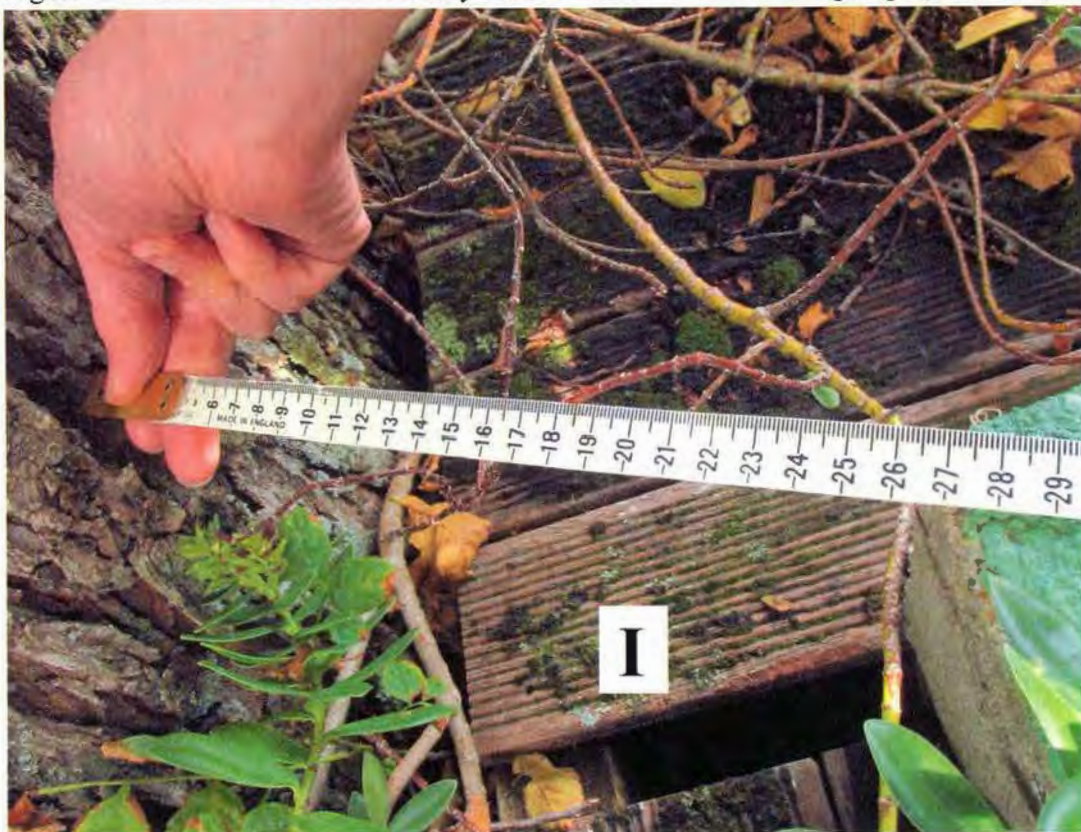
Figure 12. The elm tree's trunk is very close to the back wall of the garage (location I)
