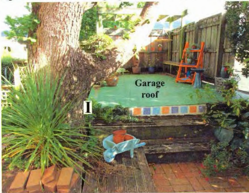
Figure 11. Roof of detached garage next to the elm tree
