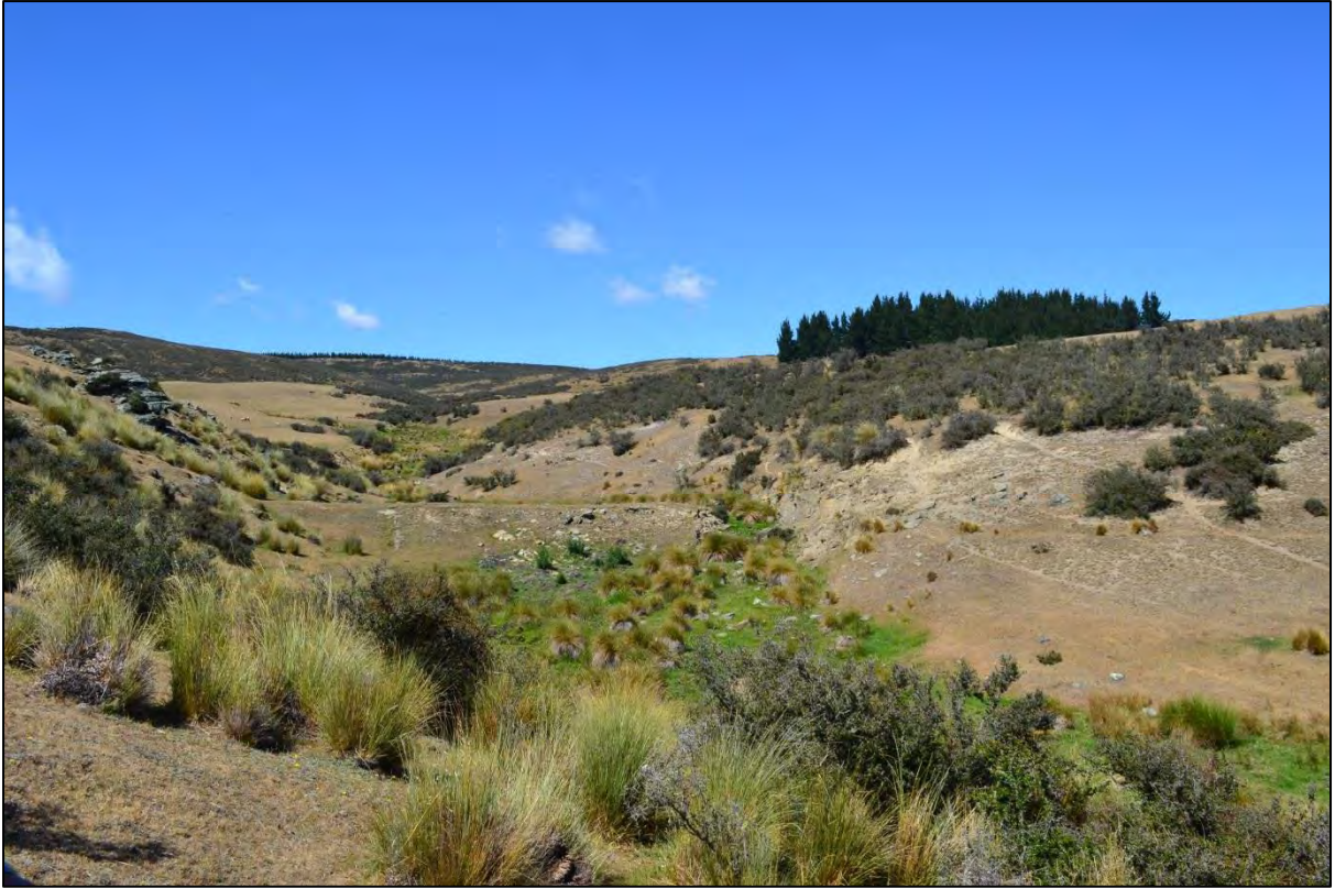
Figure 23. Dam in the distance with water-race on hillside to the right (Photo No. 5).
