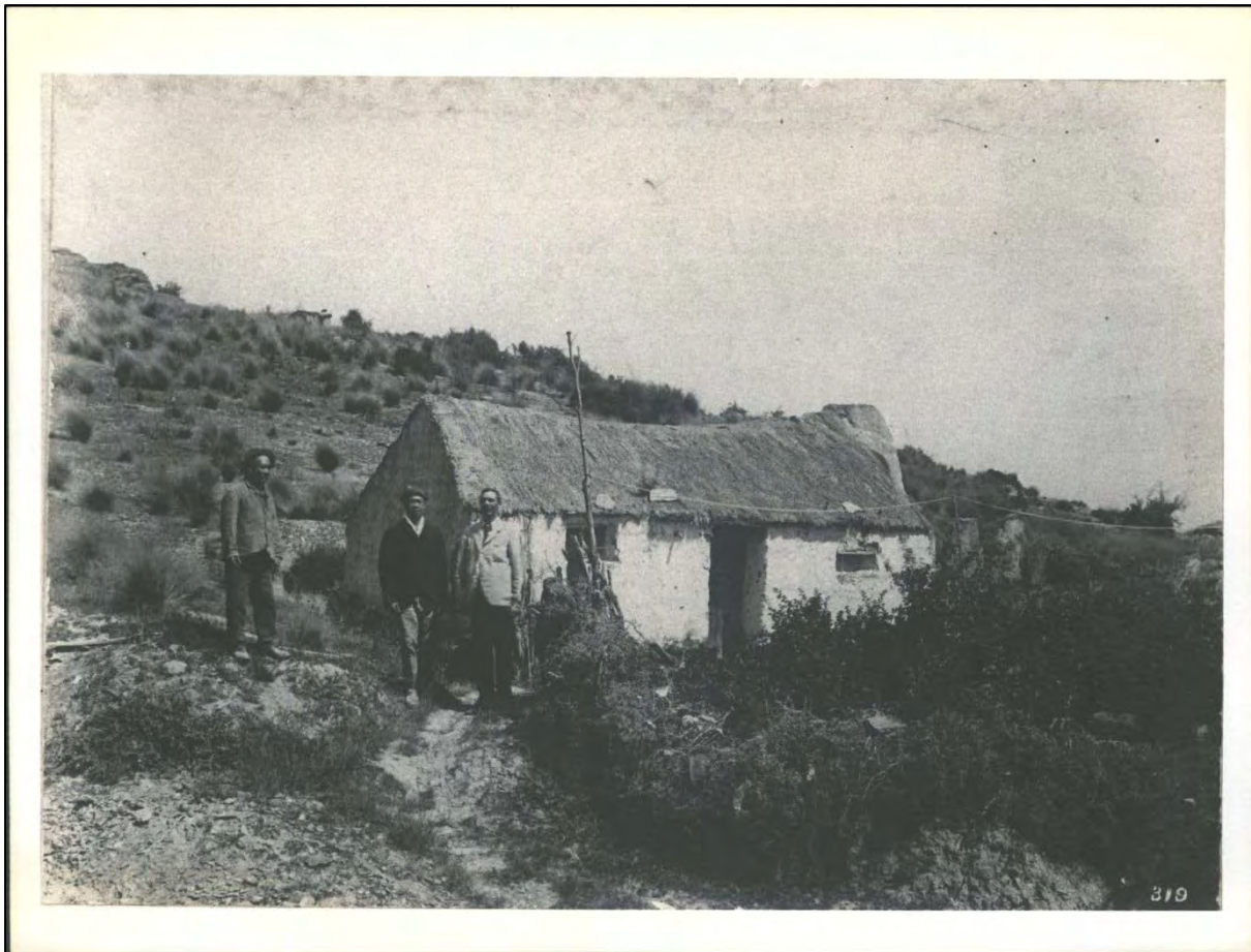
Figure 6. Goldmining at 4 Mile Creek, Fullarton. The cottage in the picture is likely to be representative of the type constructed by miners in the wider area (Hocken Snapshot).
