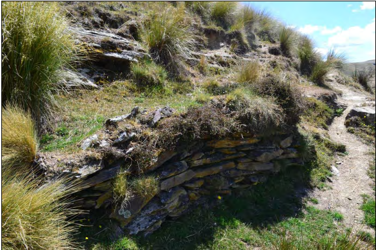
Figure 35. Stone revetment for water-race (Photo No. 14).
