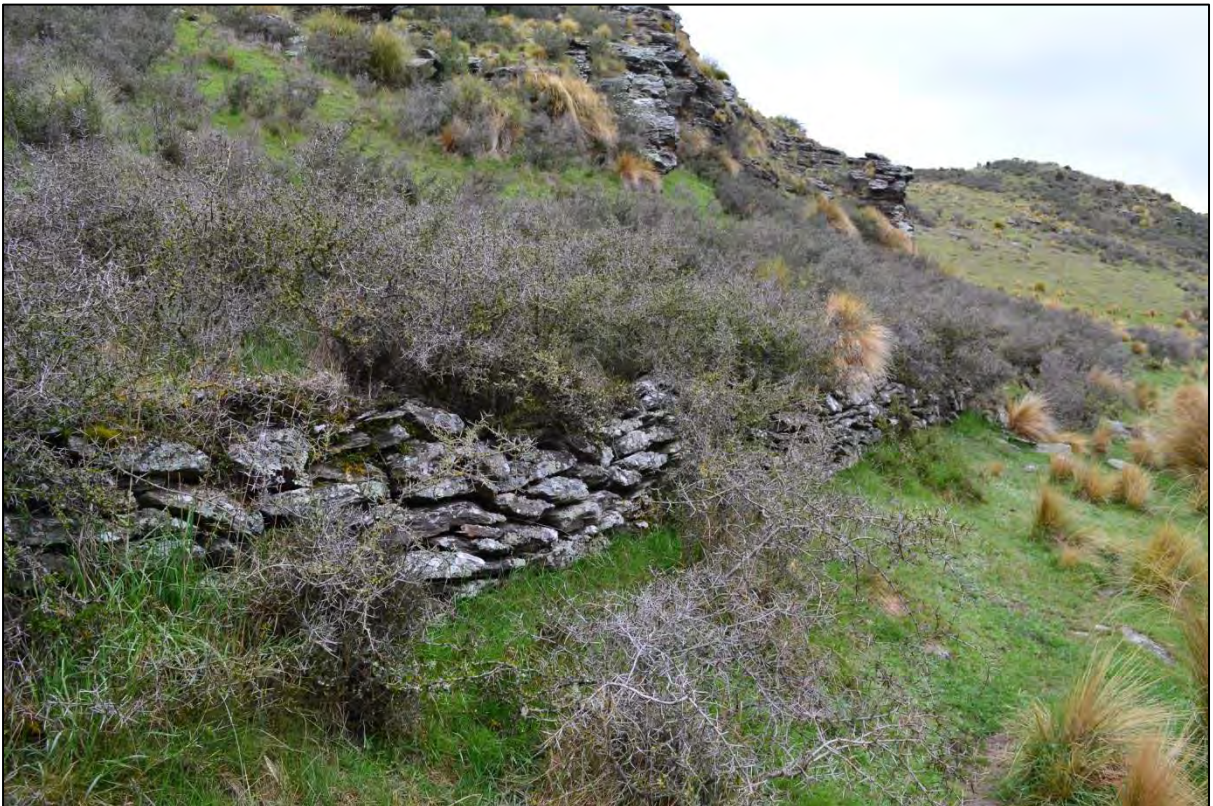
Figure 26. Stone revetting for tramline along Coal Creek (Photo No. 8).
