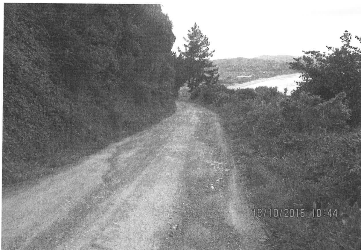
Photo 20: The section of Lyders Road the applicant proposes to upgrade. The house of 103 Cliffs Road is out of sight on the right, below the large tree in the centre of the photo.
