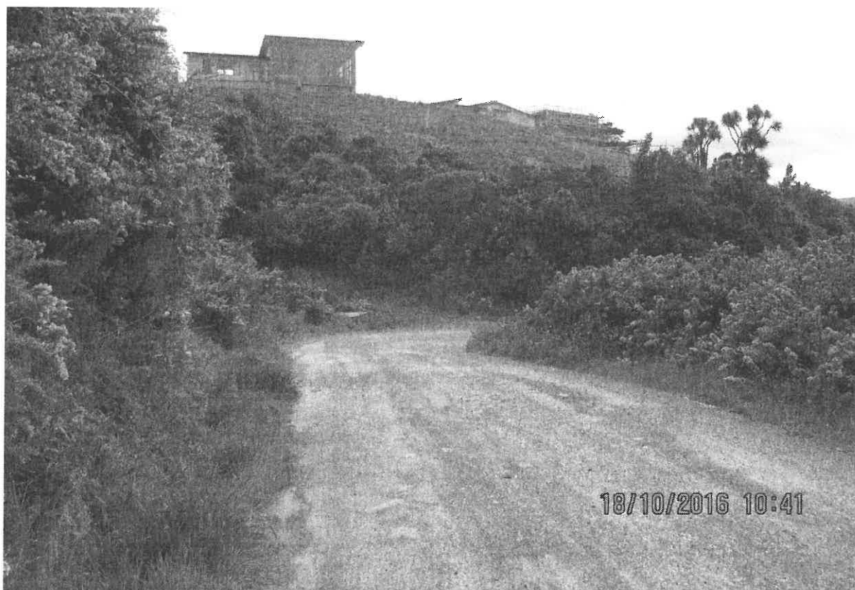
Photo 16: The bend into 101A Cliffs Road from above. The house is on 4B Clayton Street. The houses of 2F and 2G Cliffs Road will be constructed in front of this house.
