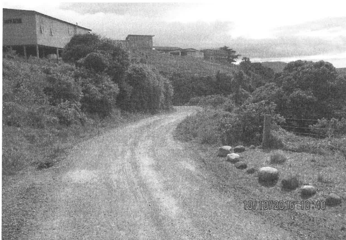
Photo 15: Looking down the Lyders Road section of the access, with 2E Cliffs Road on the left and the undeveloped land of 2F to 2L Clayton Street on the hillside.
