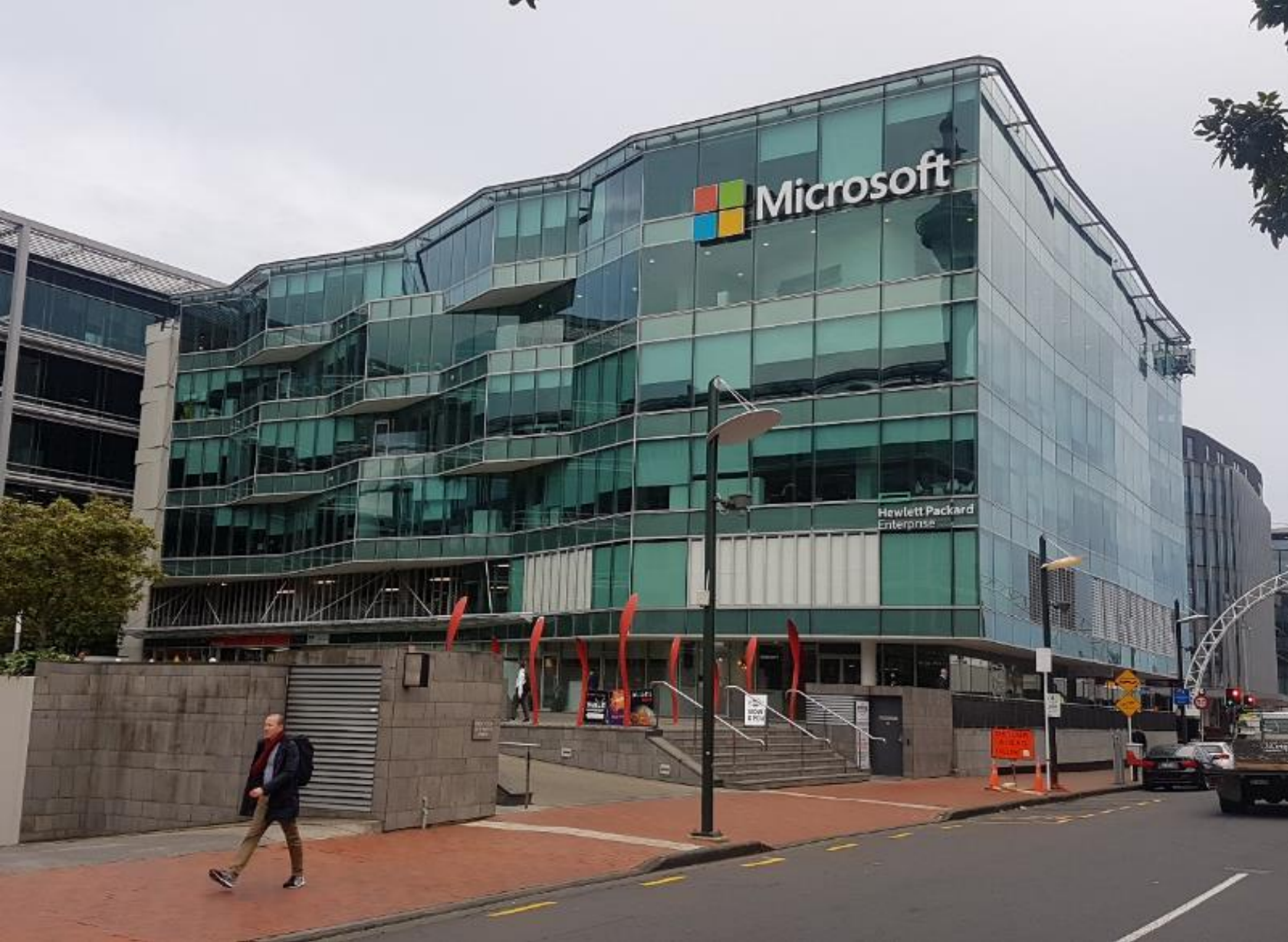
Figure 4: Example of the effect of visual weight of light green tinted vision glazing on a 6 storey building
