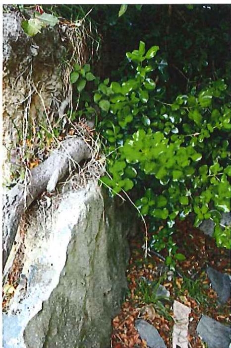
Tree roots grown through retainer wall in neighbours section
