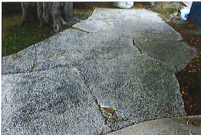
Sloping car park area and footing for extension ladder to access gutter (1 ¾ stories high)
