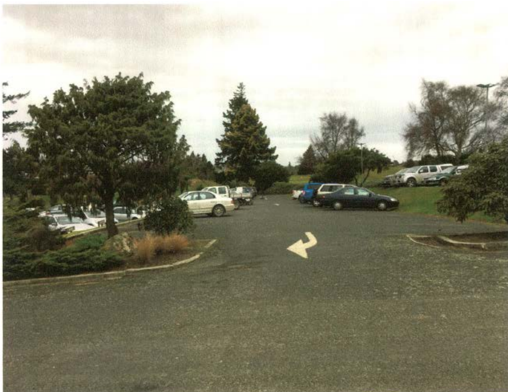
Figure D: On-site Car parking
