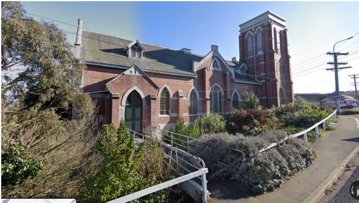
Figure 3: View from Spottiswood Street (Source – Google Maps )
