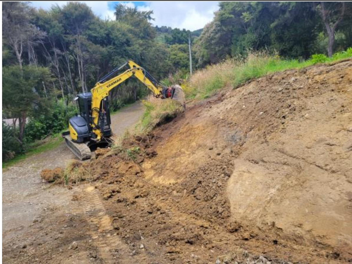
Photograph 1: Earthworks on the main (highest) cut slope underway
