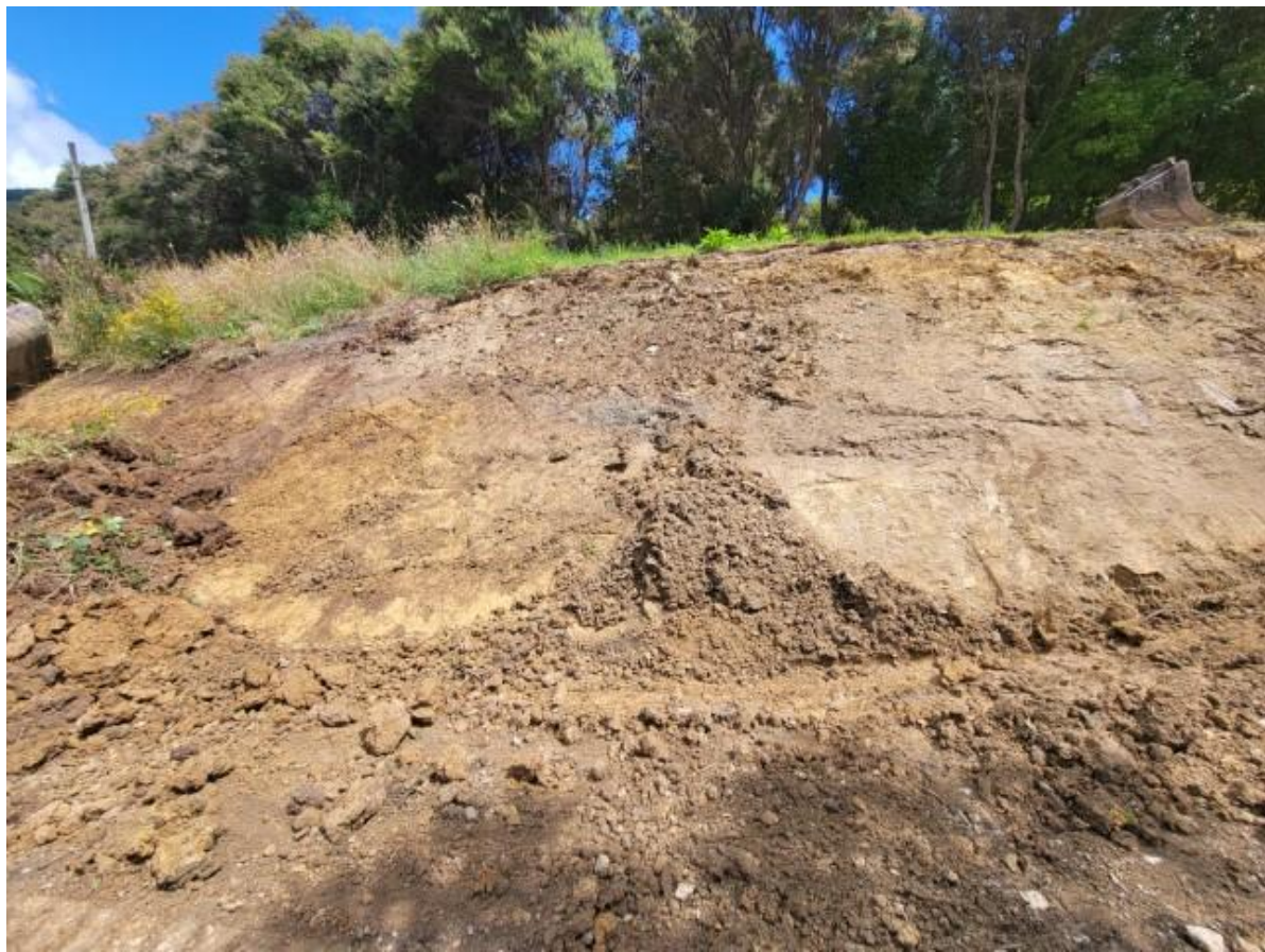
Photograph 2: Main cut slope, with the fill contact clearly visible about 1/3 of the way up the slope
