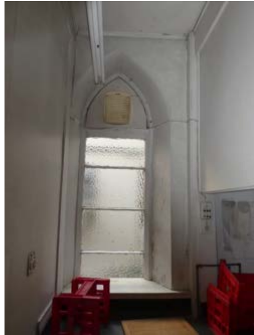
Photograph 256 – Showing the extract ventilation fan in the basement kitchen.
