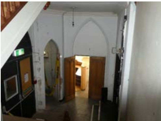
Photograph 71 - Showing the north western vestibule / stage left.
