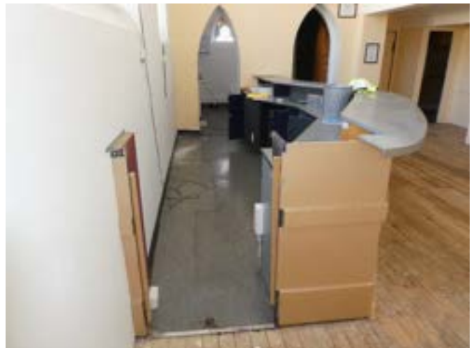
Photograph 138 – Showing vinyl flooring to the bar and kitchen area.
