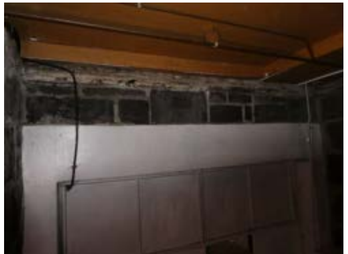
Photograph 187 – Showing the painted windows within the south western stairwell.
