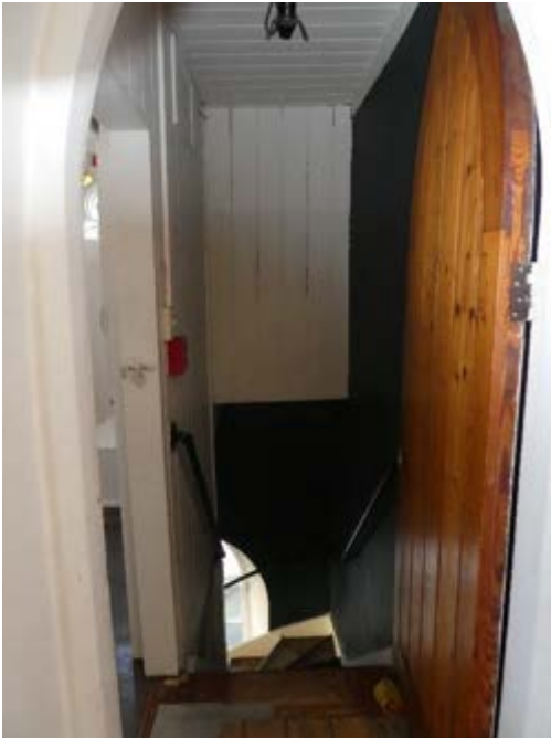
Photograph 162 - Showing the painted T&G panelling to the south western stairwell.
