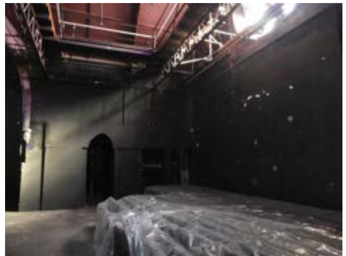
Photograph 87 – Showing the main theatre looking to the south.
