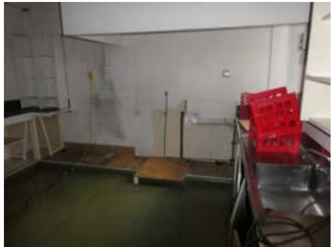
Photograph 216 – Showing the kitchen within the basement area.
