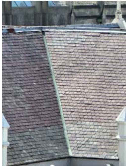
Photograph 2 – Showing the south western roofs and copper valley gutter.
