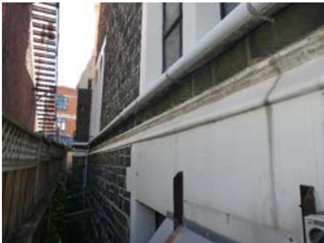
Photograph 20 – Showing the uPVC rainwater pipework to the western elevation.
