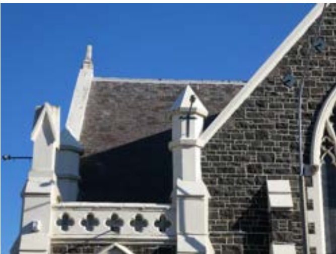
Photograph 9 - Showing the slate roof to the north eastern corner.
