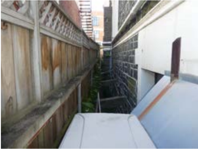
Photograph 233 - Showing the concrete braces buttressing the retaining wall to the western elevation.
