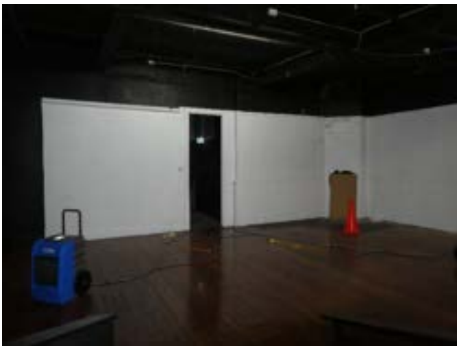
Photograph 100 - Showing the basement studio theatre space.
