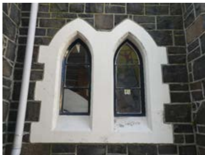
Photograph 55 – Showing the steel framed windows on the western elevation.
