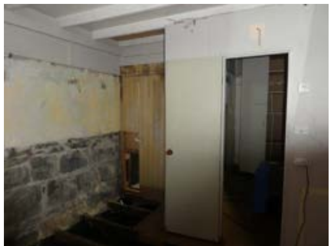
Photograph 109 – Showing the unlined / plastered walls to Dressing Room 2 accessed off the Green Room.
