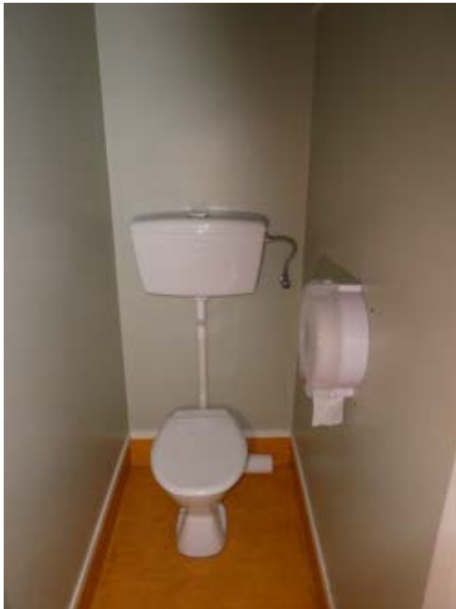
Photograph 226 – Showing the cubicle to the female toilet.
