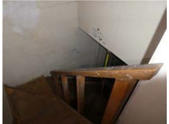
Photograph 212 – Showing the timber stairs to the south western stairwell.
