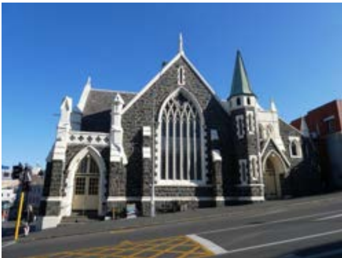
Photograph 24 - Showing the eastern elevation.
