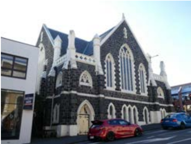
Photograph 22 - Showing the south western elevations.
