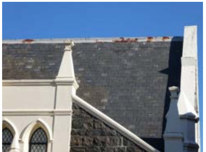
Photograph 10 – Showing the slate roof to the north western corner.
