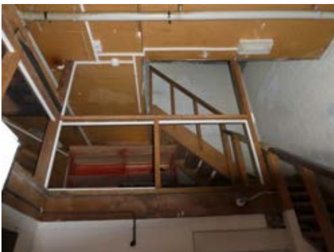
Photograph 209 - Showing the open tread stairs to the south western stairwell.
