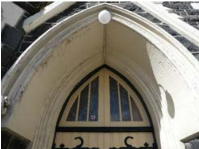
Photograph 46 - Showing the glazed top light above the northern entrance door.
