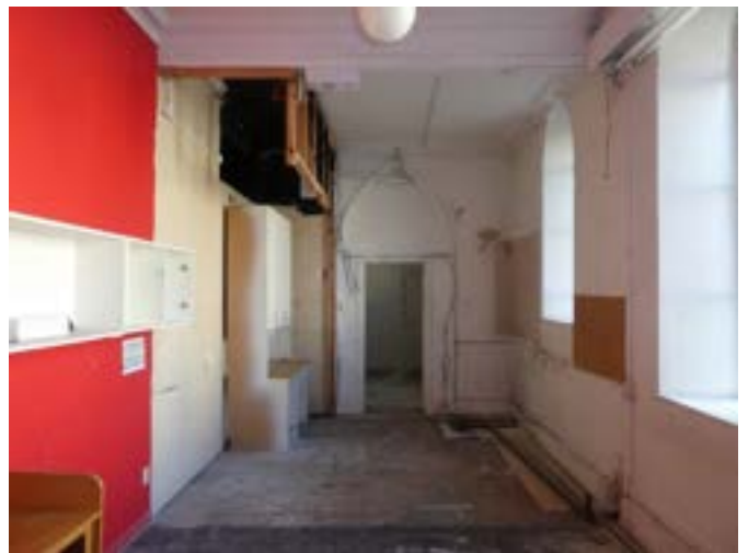
Photograph 97 – Showing the basement offices.
