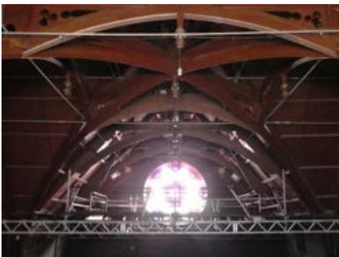
Photograph 82 - Showing the rose window looking west
