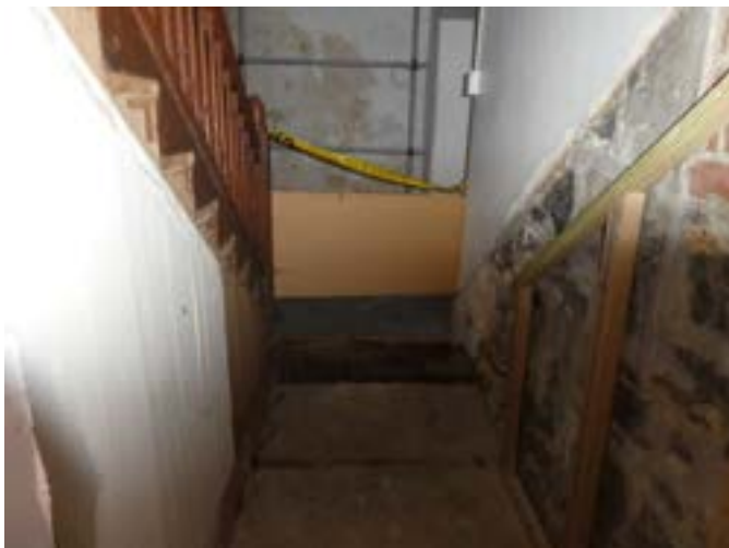
Photograph 201 - Showing the linings removed from the basement floor to the former project managers office / stairs at the north western stairwell.
