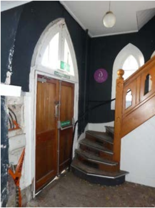
Photograph 92 - Showing the south eastern entrance and vestibule.
