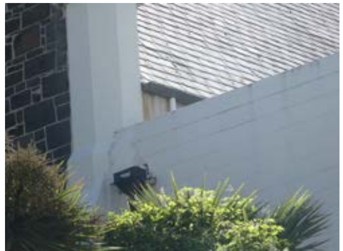
Photograph 40 – Showing the two-story extension to the south western corner.
