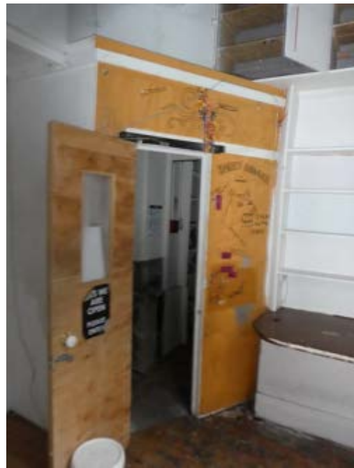
Photograph 111 – Showing the Operations Managers Office.
