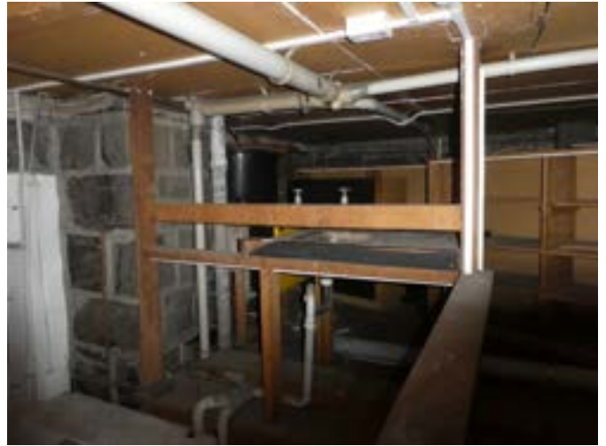
Photograph 127 – Showing the storage area above the south western toilets.
