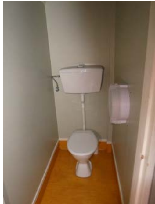
Photograph 227 – Showing the cubicle to the female toilet.
