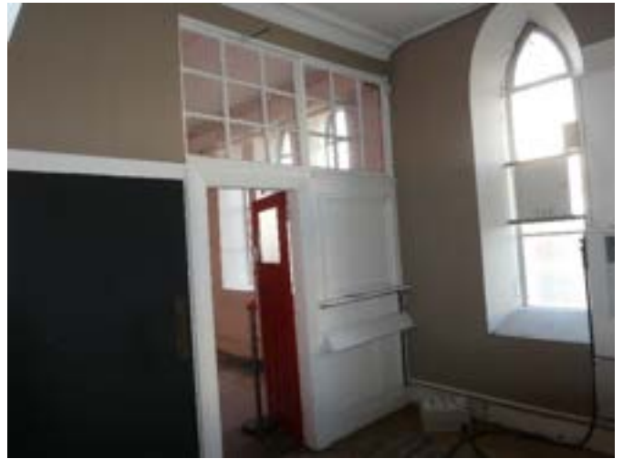
Photograph 95 – Showing the entrance to the basement offices.
