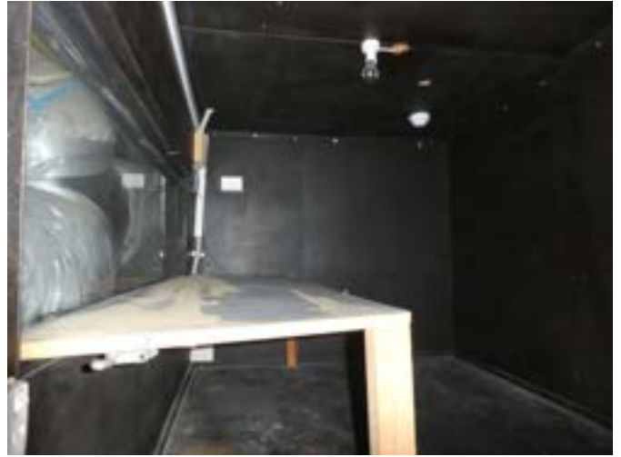
Photograph 105 – Showing the storage area / control room above the Green Room kitchen, accessed via ladder.
