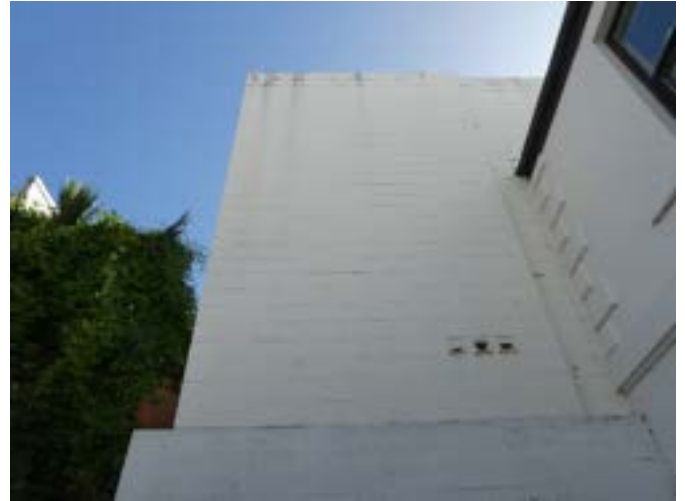
Photograph 42 – Showing the two-story extension to the south western corner.
