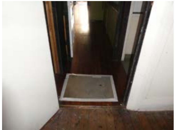
Photograph 144 – Showing the patched flooring / underfloor access outside of the Green Room.
