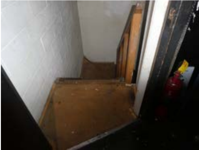
Photograph 211 - Showing the timber stairs to the south western stairwell.
