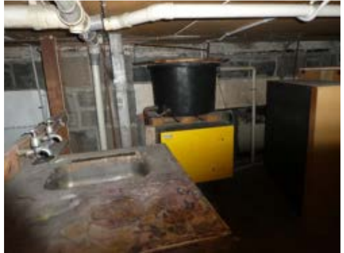
Photograph 263 – Showing the foul water pipework in the south western stairwell. Noting disconnected pipework which requires further investigation.
