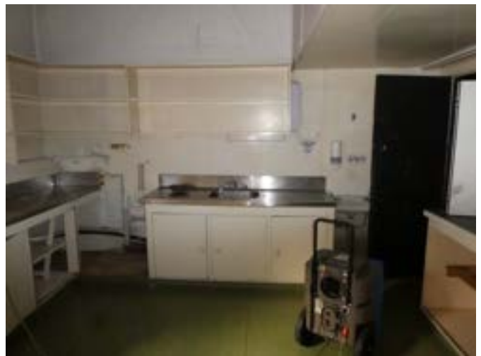
Photograph 218 – Showing the kitchen within the basement area.
