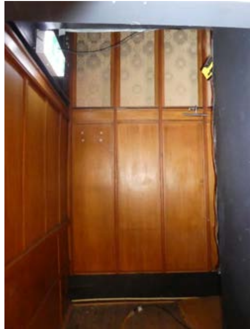
Photograph 163 – Showing the painted T&G panelling to the south western stairwell.
