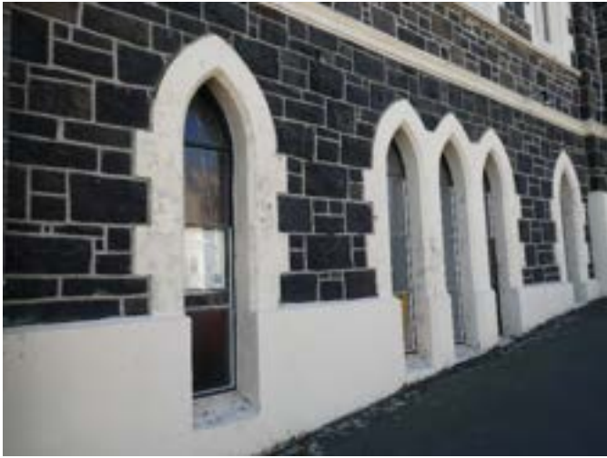
Photograph 58 - Showing the steel framed windows on the southern elevation.
