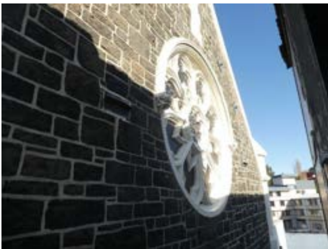
Photograph 62 - Showing the rose window to the western elevation.
