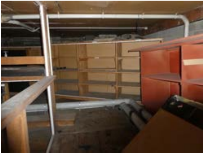
Photograph 126 - Showing the storage area above the south western toilets.
