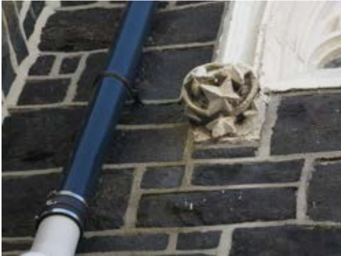
Photograph 28 - Showing typical boss detail to the windows.
