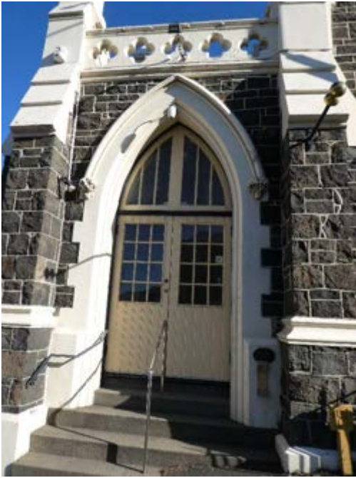
Photograph 44 - Showing the north eastern double entrance doors.
