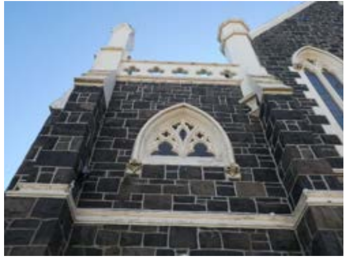
Photograph 59 – Showing the tracery window on the southern elevation.
