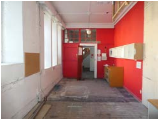
Photograph 98 - Showing the basement offices.
