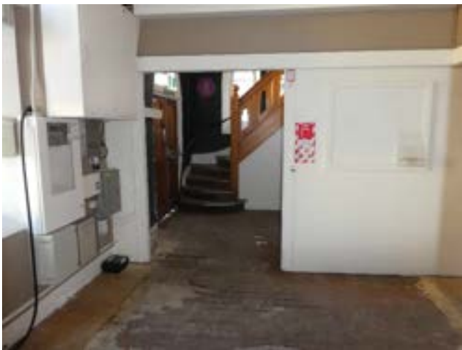
Photograph 96 - Showing the lobby to the basement theatre, toilets and offices..
