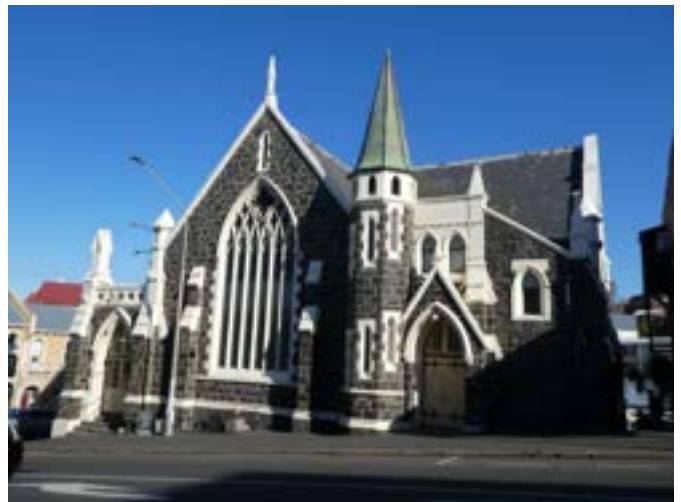
Photograph 25 – Showing the eastern elevation.
