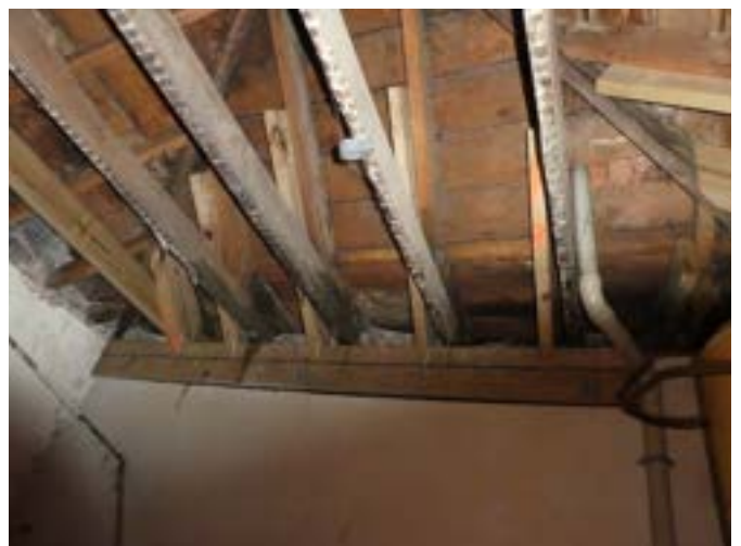
Photograph 68 – Showing the original ceiling joists and strengthening works to the rafters within the roof space above the kitchen / bar
