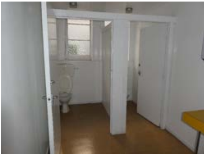
Photograph 231 - Showing the cubicles to the female toilet.
