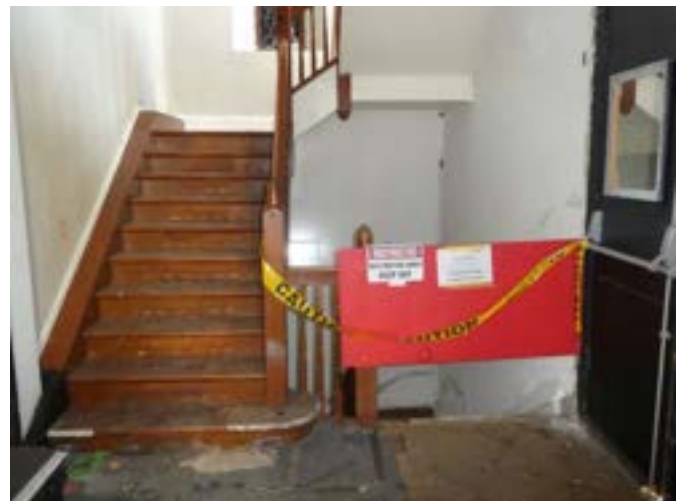
Photograph 72 – Showing the staircase from the north western vestibule / stage left.
