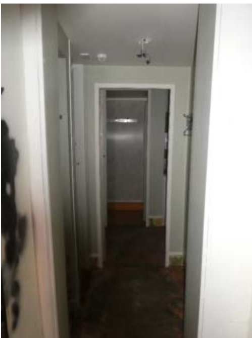
Photograph 222 – Showing the lobby to the shower and the female toilets.
