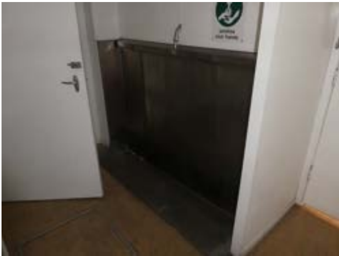
Photograph 229 - Showing the urinal to the male toilet.
