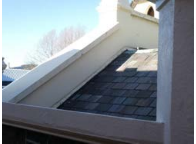
Photograph 12 – Showing the flashings detail to the rear of the parapet wall to the north western corner.
