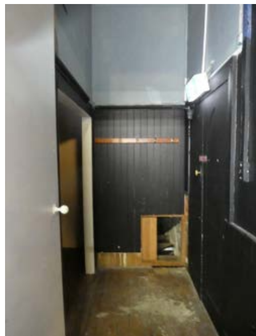
Photograph 148 – Showing original painted timber panelling to the basement area.
