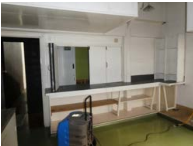
Photograph 217 - Showing the kitchen within the basement area.
