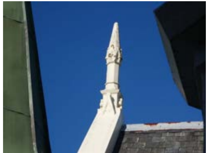
Photograph 27 – Showing the pinnacle to the northern gable.
