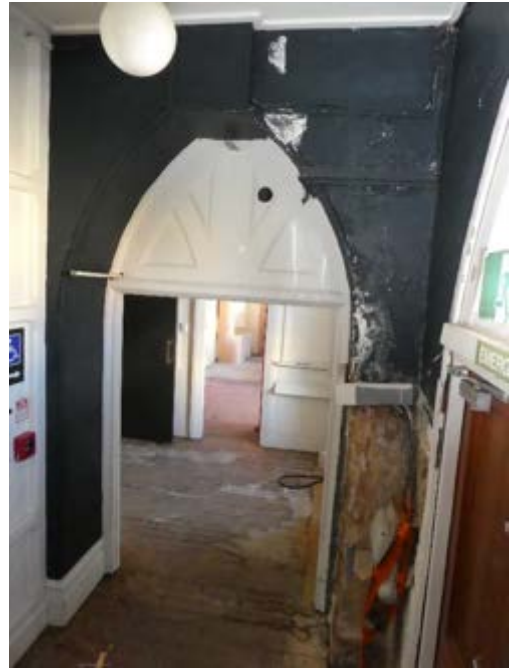
Photograph 93 – Showing the south eastern entrance and vestibule.
