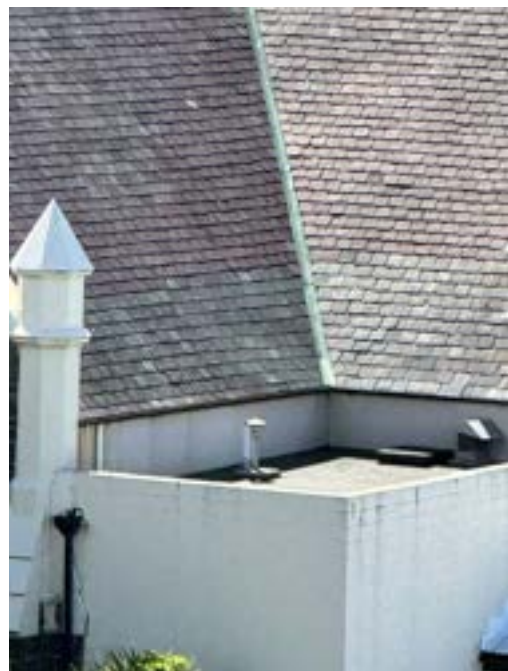
Photograph 14 – Showing the south western roofs and flat roof area above the extension.
