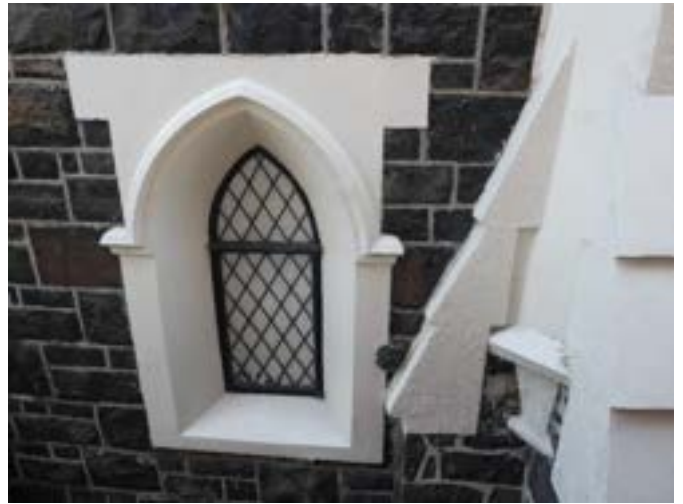
Photograph 61 – Showing the leadlight lancet window and buttress to the north eastern elevation.
