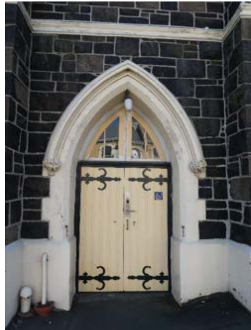
Photograph 43 – Showing the south western double entrance doors.
