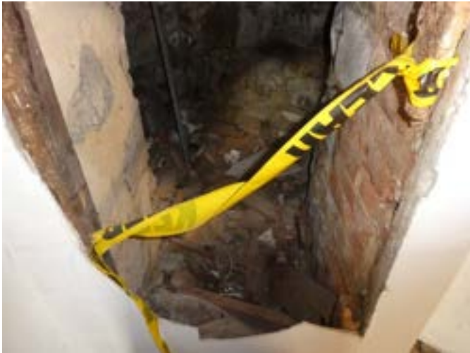
Photograph 160 - Showing the bell tower / turret from within the basement area.
