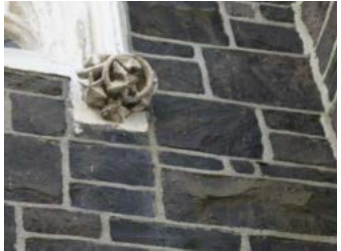
Photograph 29 – Showing typical boss detail to the windows.
