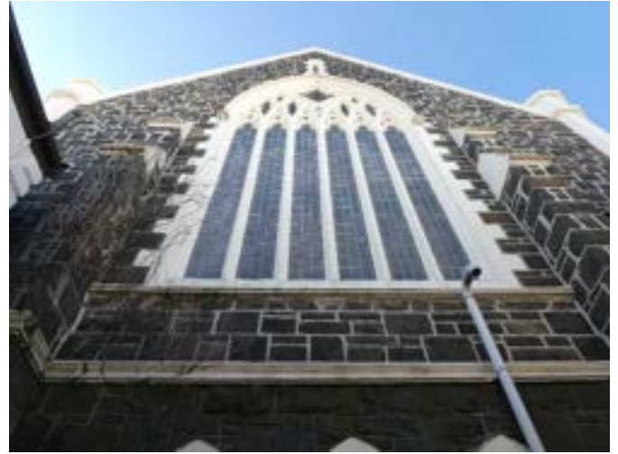
Photograph 49 – Showing the southern tracery window.
