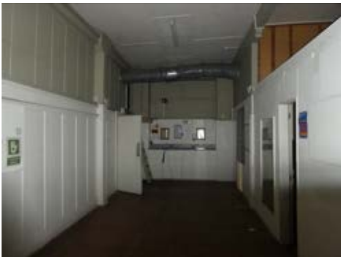
Photograph 102 - Showing the Green Room and kitchenette behind the basement studio theatre. The upper levels appear to be the original glazing which has been painted.
