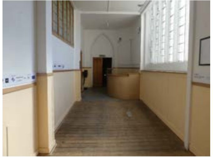
Photograph 74 – Showing the reception desk and main entrance foyer.
