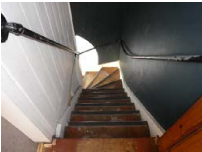
Photograph 213 - Showing the timber stairs to the south eastern stairwell.
