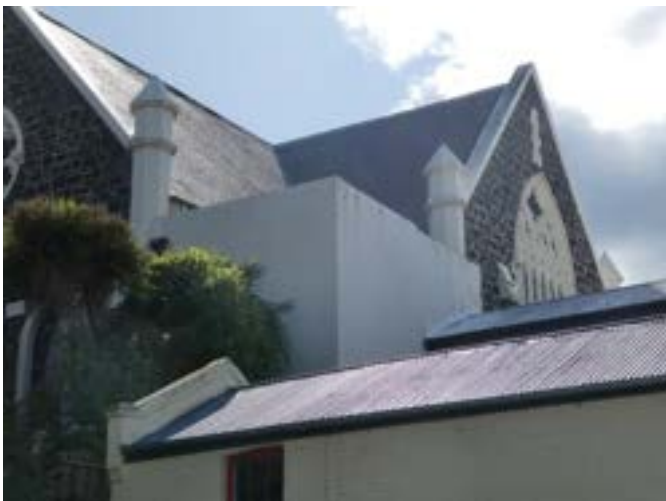
Photograph 39 – Showing the two-story extension to the south western corner.
