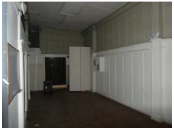
Photograph 103 – Showing the Green Room behind the basement studio theatre. The upper levels appear to be the original glazing which has been painted.
