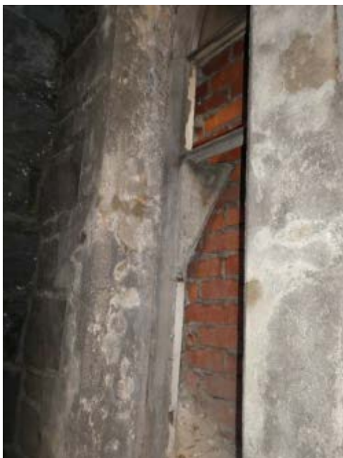
Photograph 50 - Showing the broken glazing to the steel framed windows which has been bricked up to the south western courtyard area.
