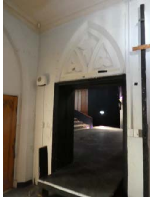
Photograph 189 – Showing the double entry door to stage left from the north western vestibule.
