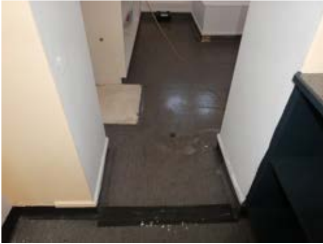
Photograph 139 - Showing vinyl flooring to the bar and kitchen area.
