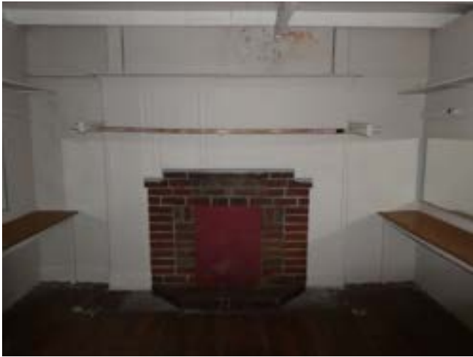
Photograph 106 - Showing the blocked up fire place within Dressing Room 1 accessed off the Green Room.
