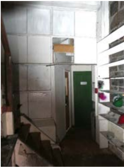
Photograph 110 – Showing the south western stairwell looking to the Operations Managers Office.
