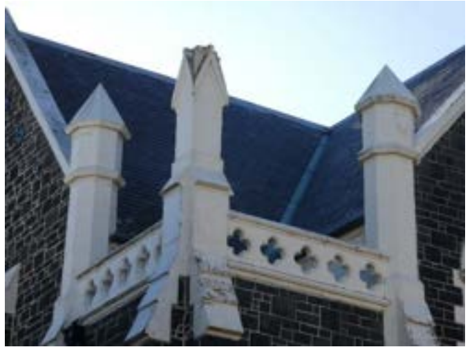
Photograph 8 – Showing the slate roof to the south eastern corner.
