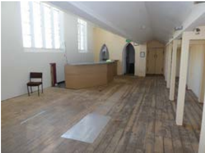
Photograph 77 - Showing the eastern bar area.
