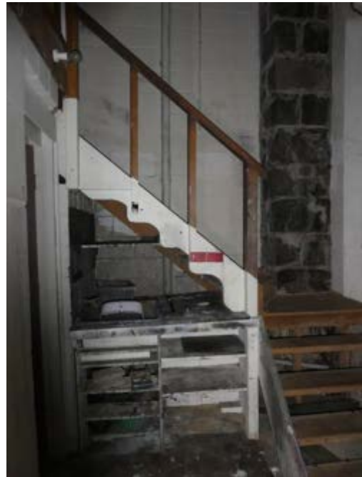
Photograph 208 – Showing the open tread stairs to the south western stairwell.
