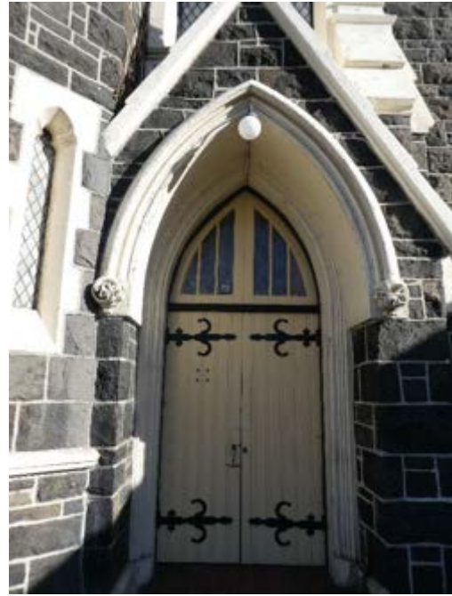
Photograph 45 – Showing the north western double entrance doors.
