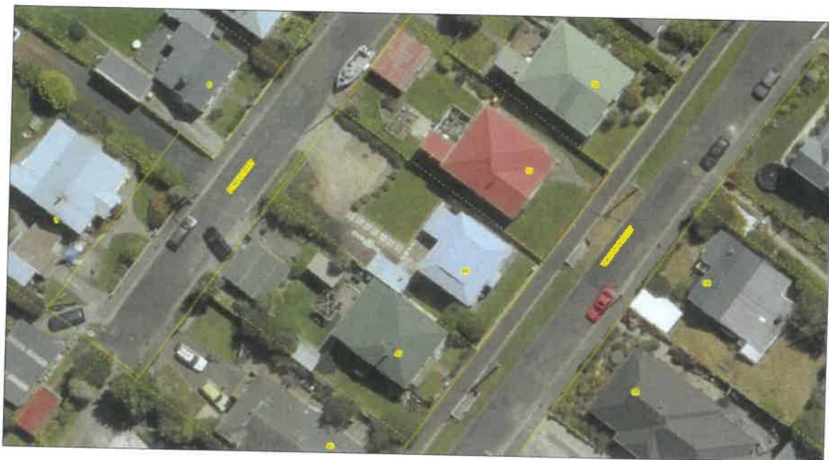
Photo A – Aerial view of application site.
