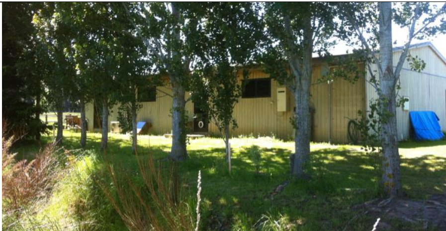
Above: Photo taken from the submitters land of the shed, highlighting the deciduous trees and the windows/doors facing the boundary.
