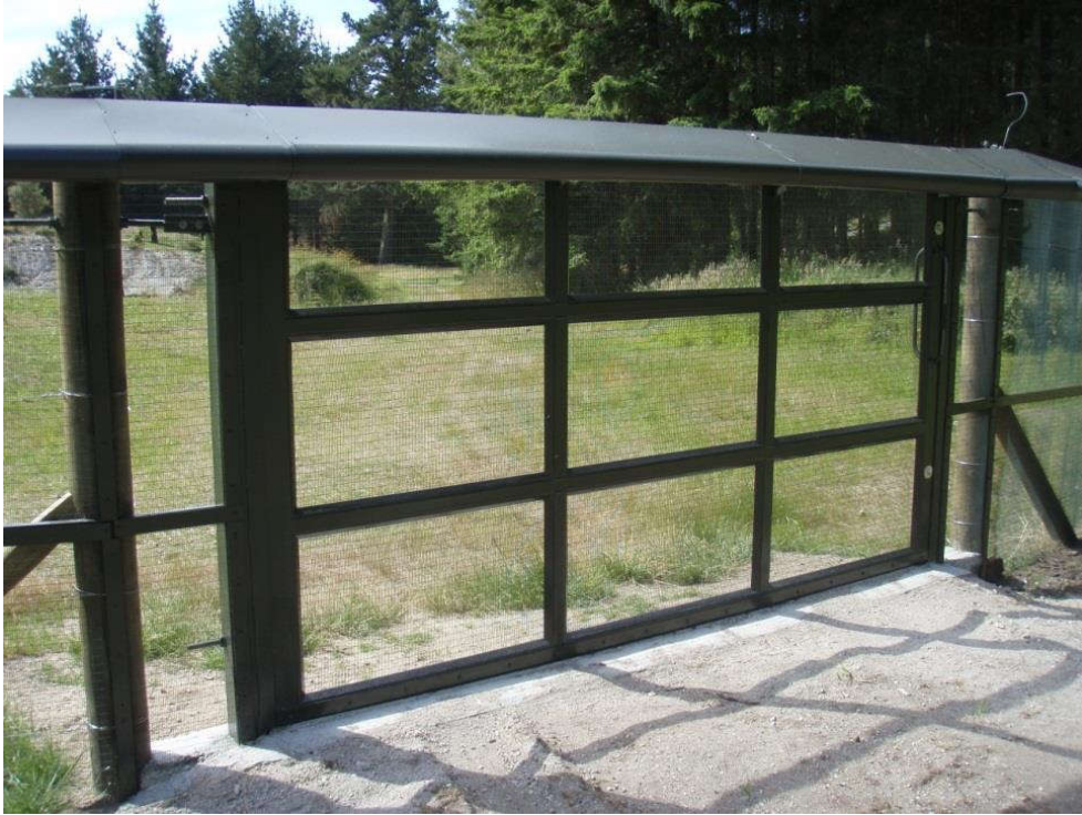
Figure 1-5: Xcluder® vehicle access gate installed in an Xcluder® “All-Pest” fence.
