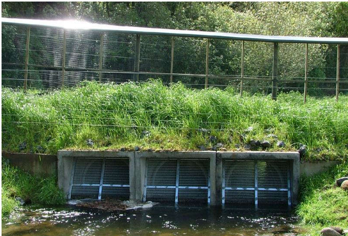
Figure 1-2: Xcluder® swinging water gates mounted in concrete box culverts.
