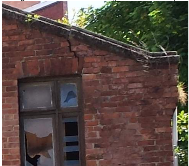
Figure 15 - Gable end wall (photo from 2013)
