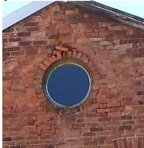
Figure 16 - Gable end wall (photo from 2013)
