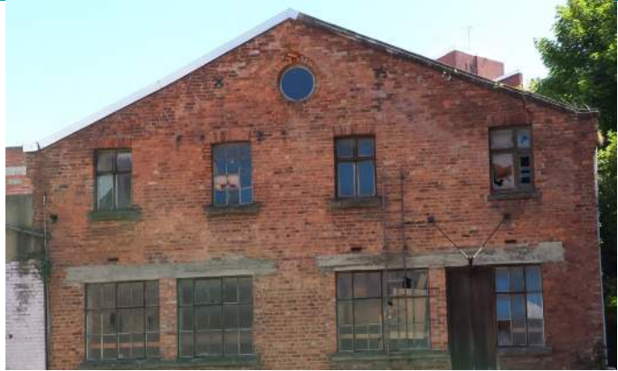
Figure 14 – Gable end wall (photo from 2013)
