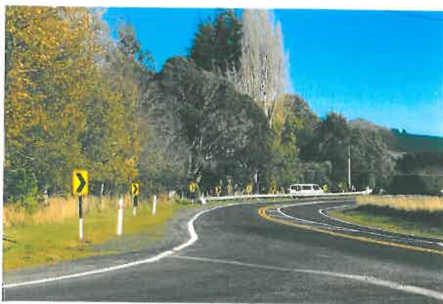
Photograph 9: Chevron Boards at the Factory Road Curve
