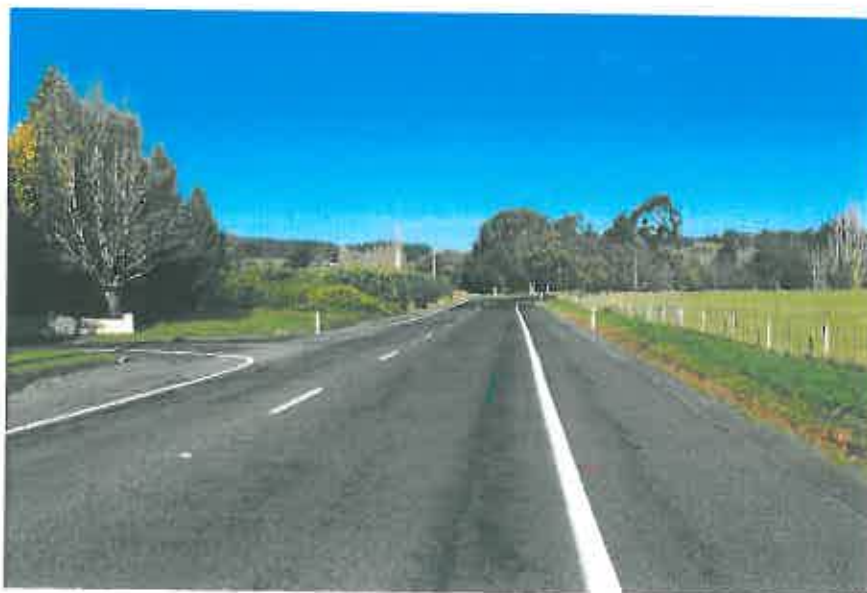
Photograph 8: Puddle Alley Looking South Towards Factory Road
