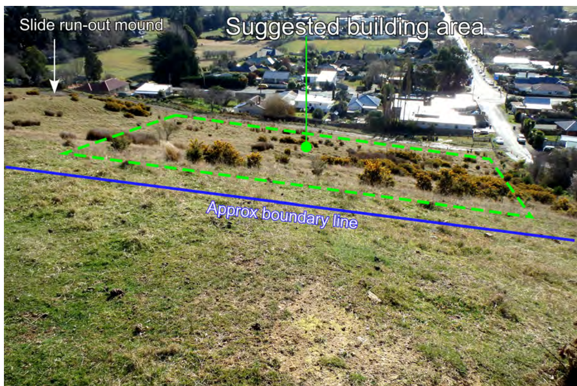
Figure 5 Northwards view of the suggested building area.
