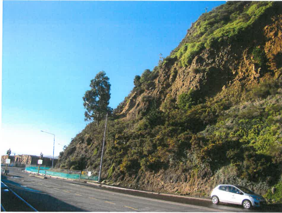
View from Beach Street towards the south east showing material to be removed and reshaped for greater safety and site geotechnical security.
