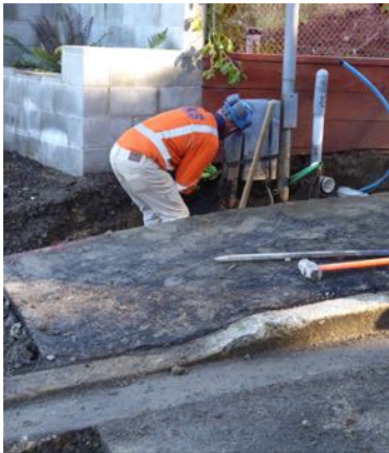
Drainage connections excavated without damaging kerbing
