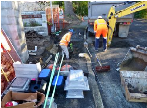
Laying drains within the TPZ of Silver Fir (T444)
