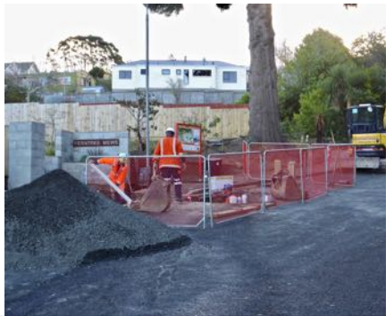
Backfill with AP20 gravel
