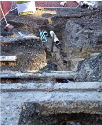
Drainage connections excavated without damaging kerbing
