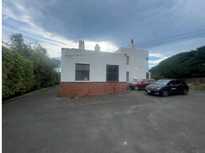
Southwest elevation showing the single storey component at the rear
