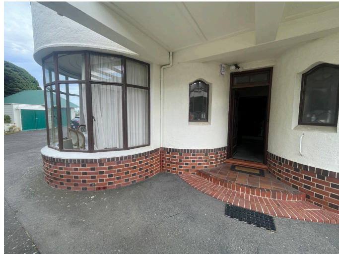
The secondary motor entrance on the northeast elevation.
