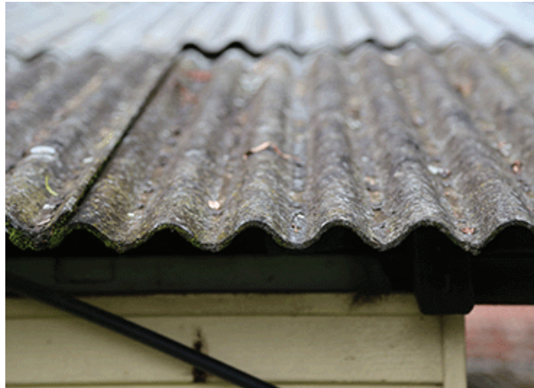
"Super Six" asbestos roof sheets
