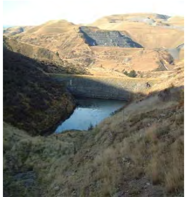
Plate 2. Deepdell North Silt Pond
