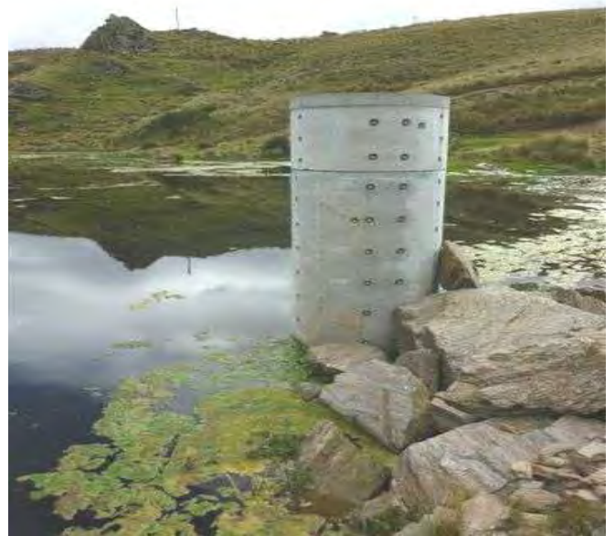
Plate 6. Typical Silt Pond Decant Structure
