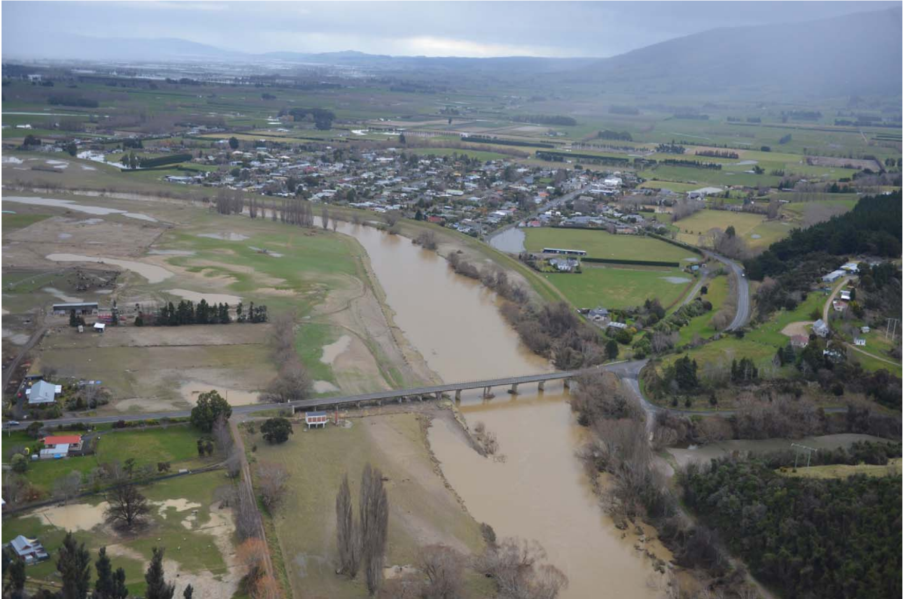
Figure 3. Taieri River in the vicinity of Outram – 25/07/2017 afternoon. The photo was taken three days after the Taieri River has peaked. Ponding is still visible on some sections of the site of interest (right bank) – Photo provided by the ODT
