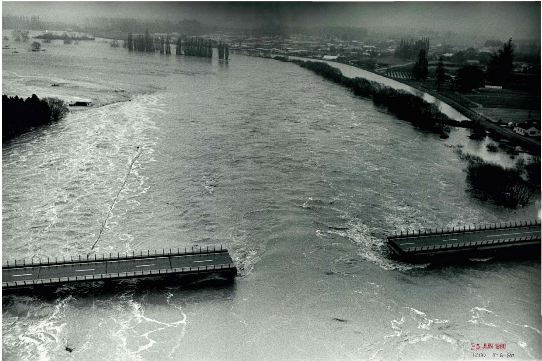
Figure 4. Outram Bridge during the June 1980 flood event. The Outram Township and the Lower Taieri Flood Protection Scheme right bank floodbank are visible at the top right corner of the photo
