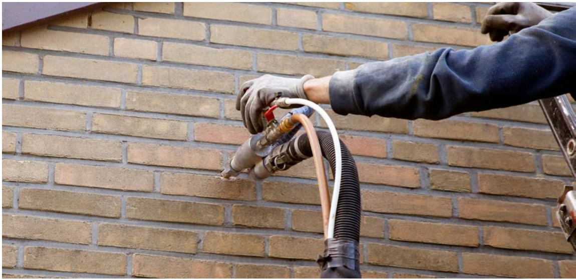
Sculptures (top left); Shade sails (top right); Injected insulation (bottom).
