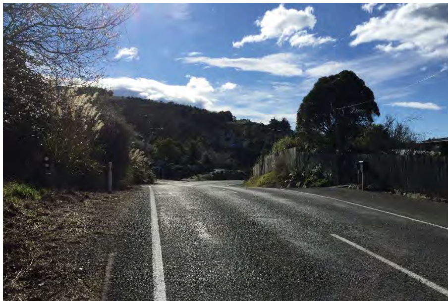
Photograph 1: Looking East Towards Perry Street from Coast Road
