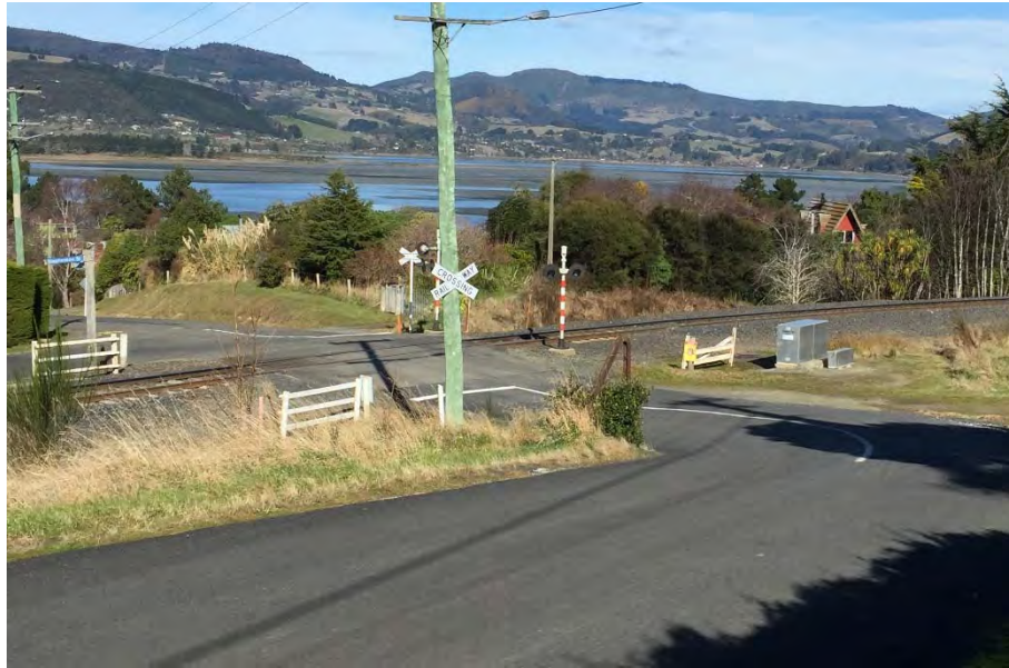
Photograph 5: Looking South Towards Curve and Railway Level Crossing
