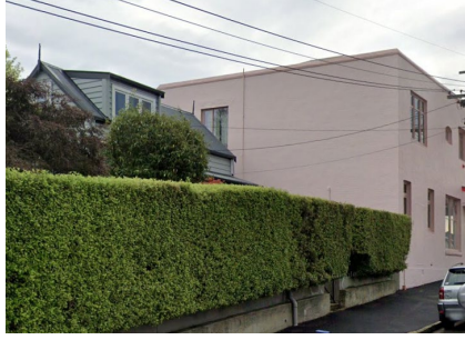
Existing south elevation from Arthur Street
