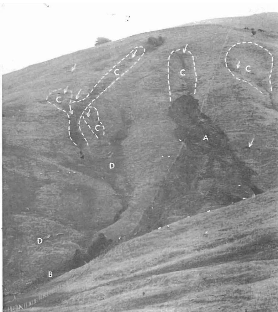
Fig.4 Debris avalanche (A) near Peggy's Hill. Flow debris (B) ex- tended 200 m down valley. Arrows locate tension cracks. Potential landslide zones (C) and old landslide debris accumulations (D) are shown.
