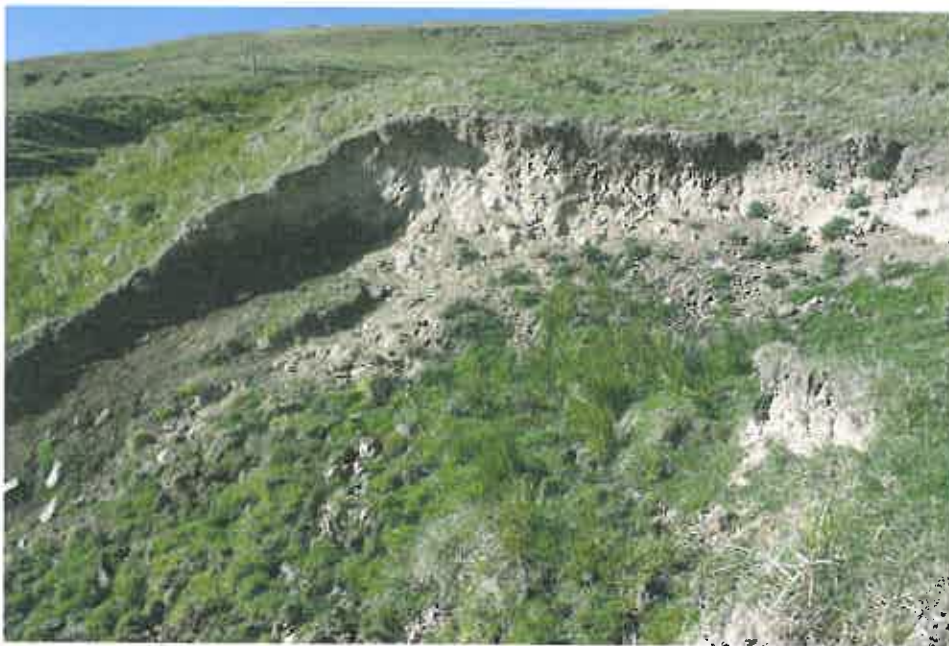
2013 landslide looking directly towards site of proposed Turbine 3 - approx 200m away
