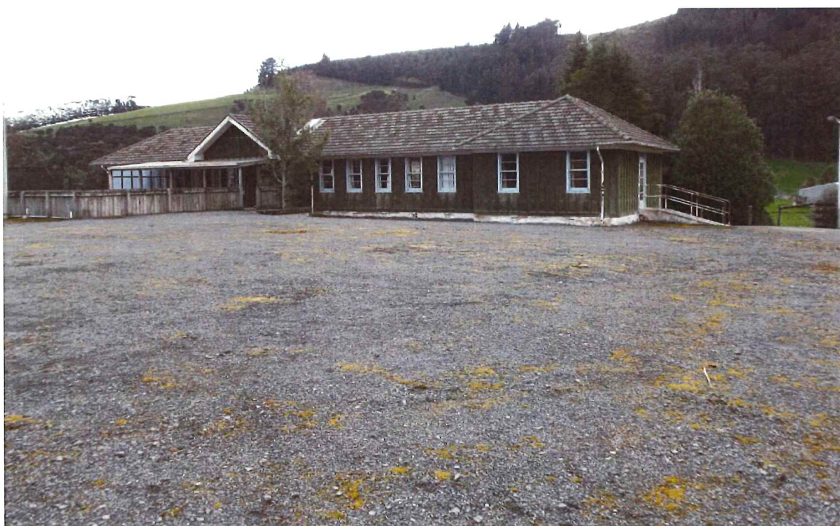
Photo 12: The villa of Lot 44, looking across the parking area of proposed Lot 41.
