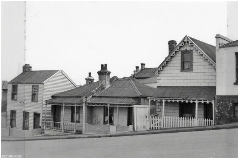
Some 'substandard' housing identified on Melville Street in the 1950s (DCC Archives, https://digitalnz.org/records/36157667/houses-in-melville-street-identified-as-substandard-in-1957 )
