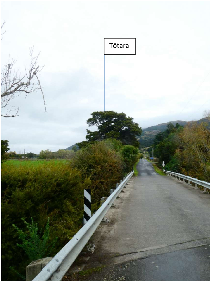
Figure 5: Totara at 125 Woodside Road
