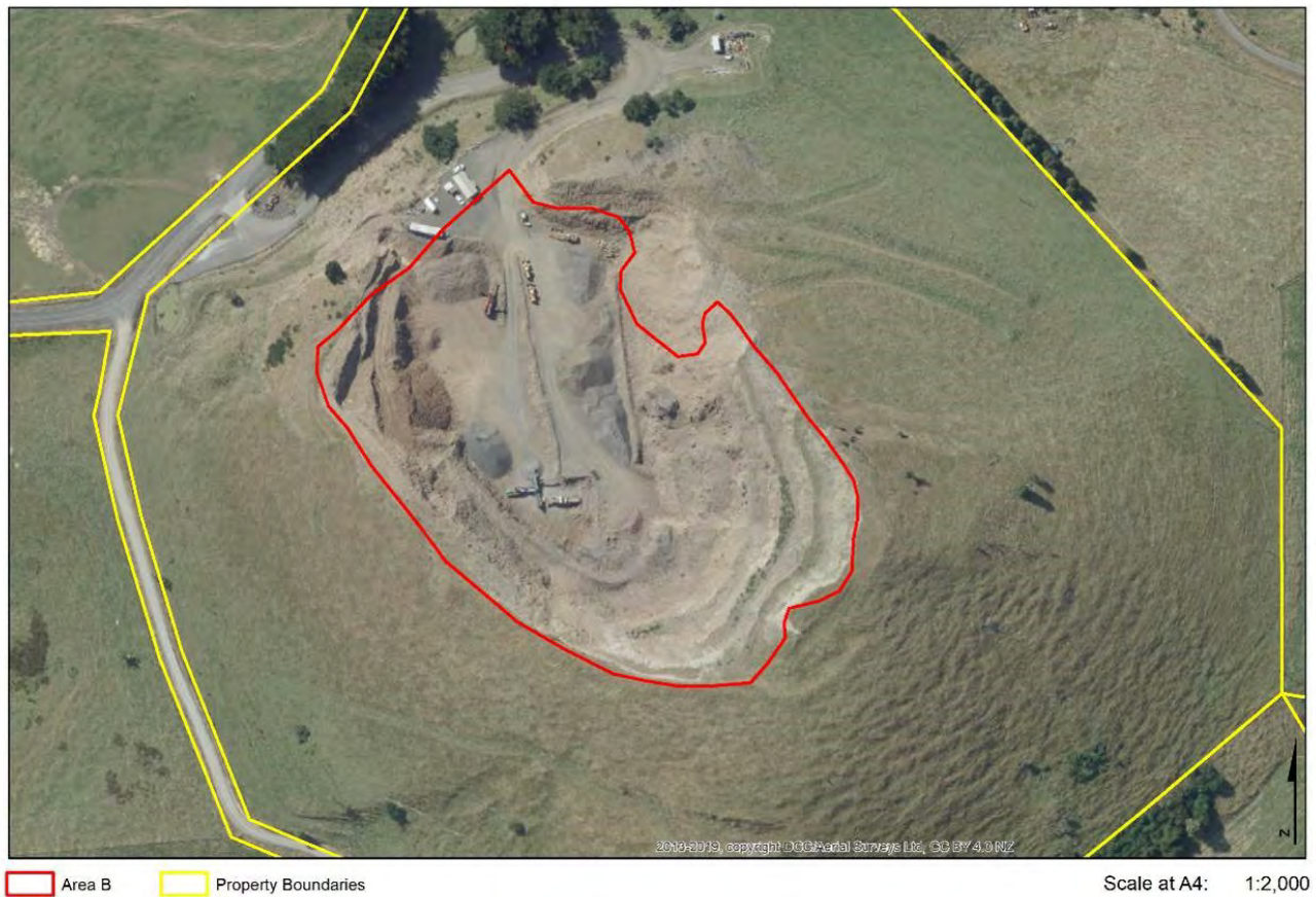
Figure 16.5.16.4B: Saddle Hill Lower Quarry: operating limits
