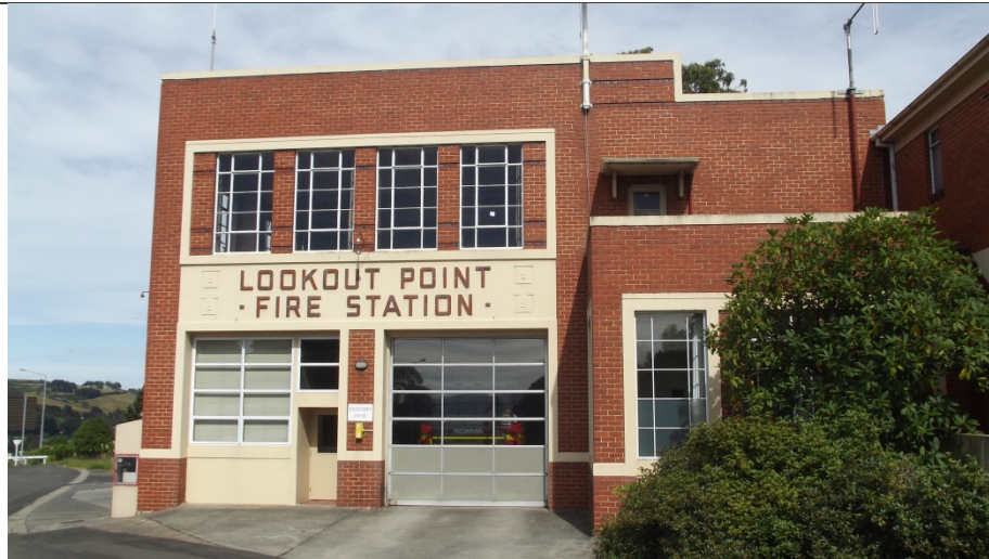
East Elevation of South Wing.
