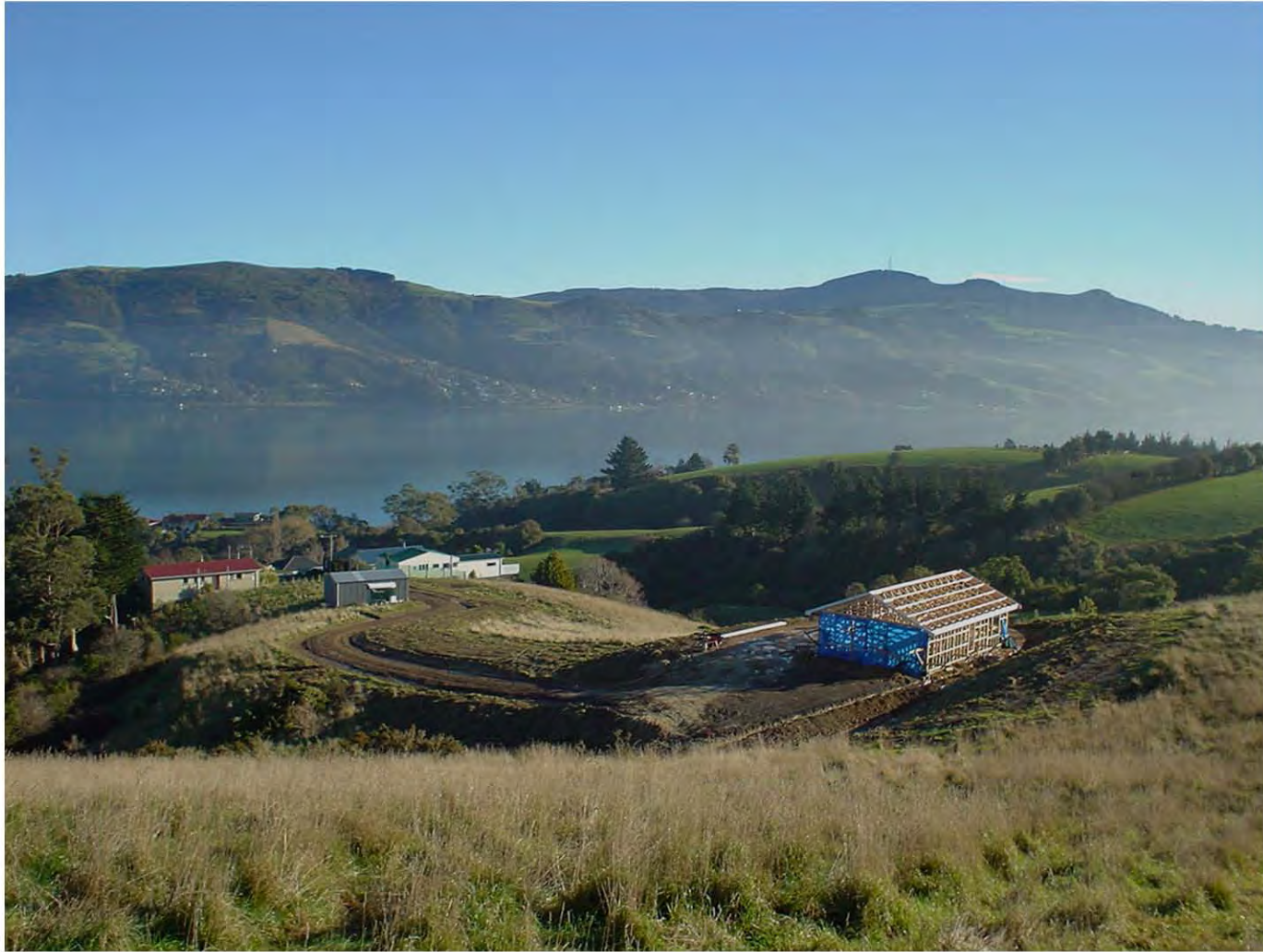
Residence @ 34 Gorman Street - 2002
