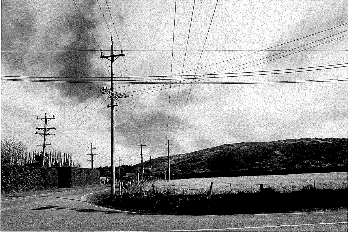
Photo 11: Looking southwest from the intersection of Huntly Road and Formby Street. Proposed Lot 1 is situated at this corner, and will be wider than the other residential lots to accommodate the two lines of power lines along the Huntly Road frontage.
