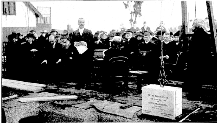
The Rev HH Barton laying the foundation stone in 1920. Otago Witness 28 September 1920, p. 32 (supplement).
