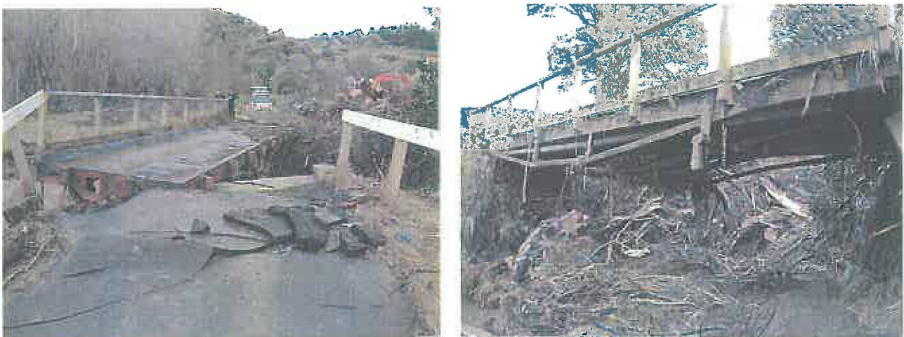
McIntosh Road Bridge
