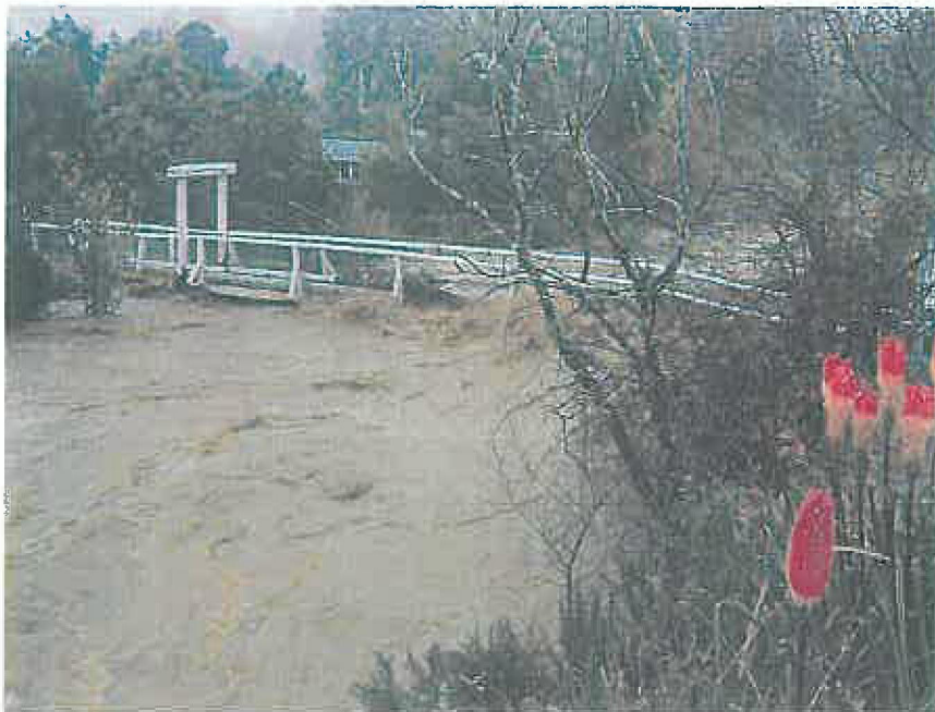
Footbridge Connecting Erne Street to Orokonui Road
