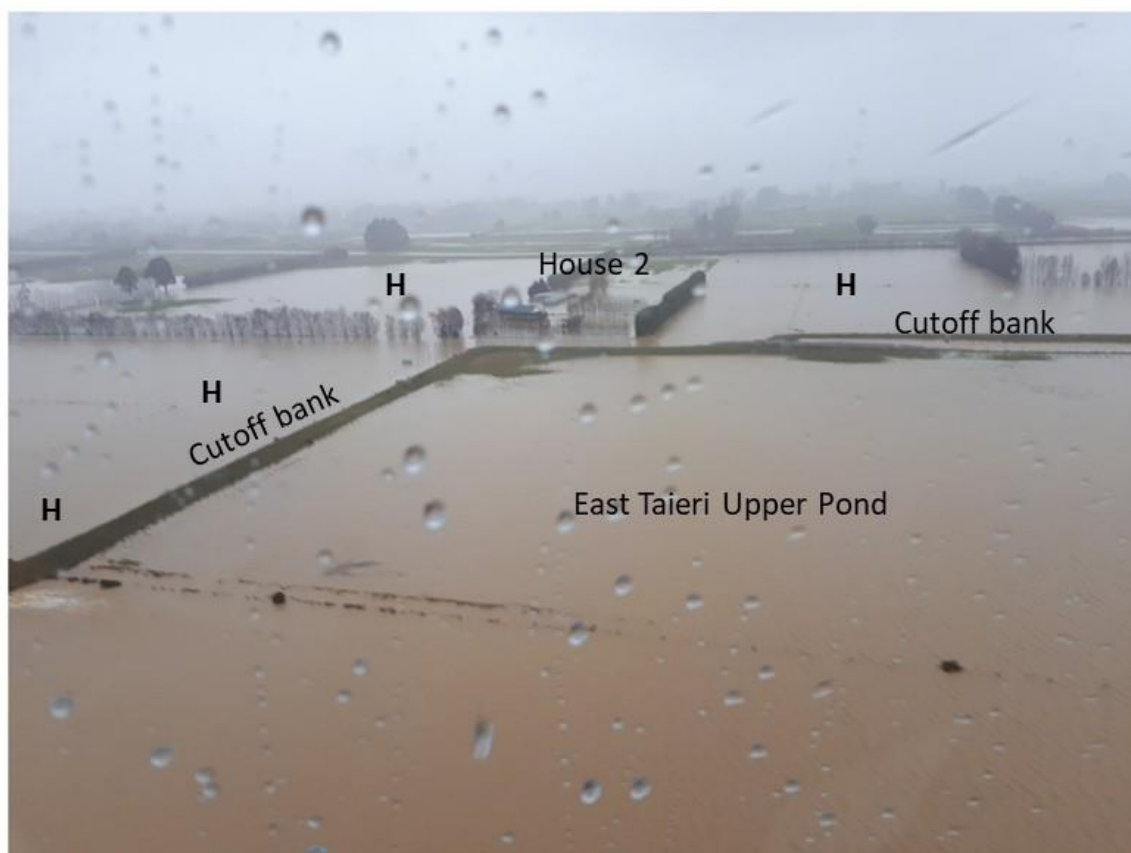
Photograph 4. Gordon Road Floodway higher risk areas (marked by "H" on the photograph) and East Taieri Upper Pond - 22 July 2017 flood event between 9am and 9.05am. House 2 showed to assist orientation
