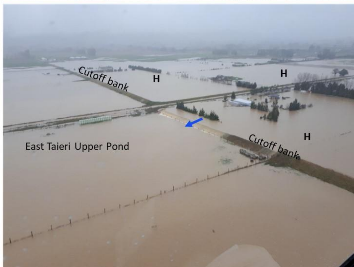
Photograph 1. Gordon Road Floodway higher risk areas (marked by "H" on the photograph) and East Taieri Upper Pond - 22 July 2017 flood event between 9am and 9.05am. Cutoff bank overtopping. The Cutoff bank is approximately 2m high at the location of the overtopping (marked with the blue arrow)
