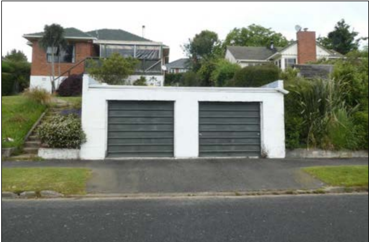
Figure 4: Houses along Mayfield Avenue with sloping frontages and garages.
