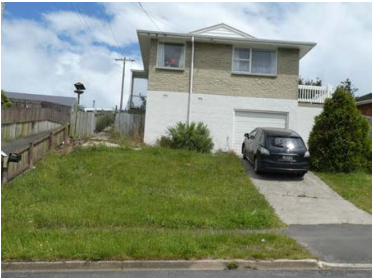
Figure 3: Typical 1:1 site ratio with a single dwelling, driveway and integral garage found commonly across the Concord assessment area (Mulford Road at Morris Street).
