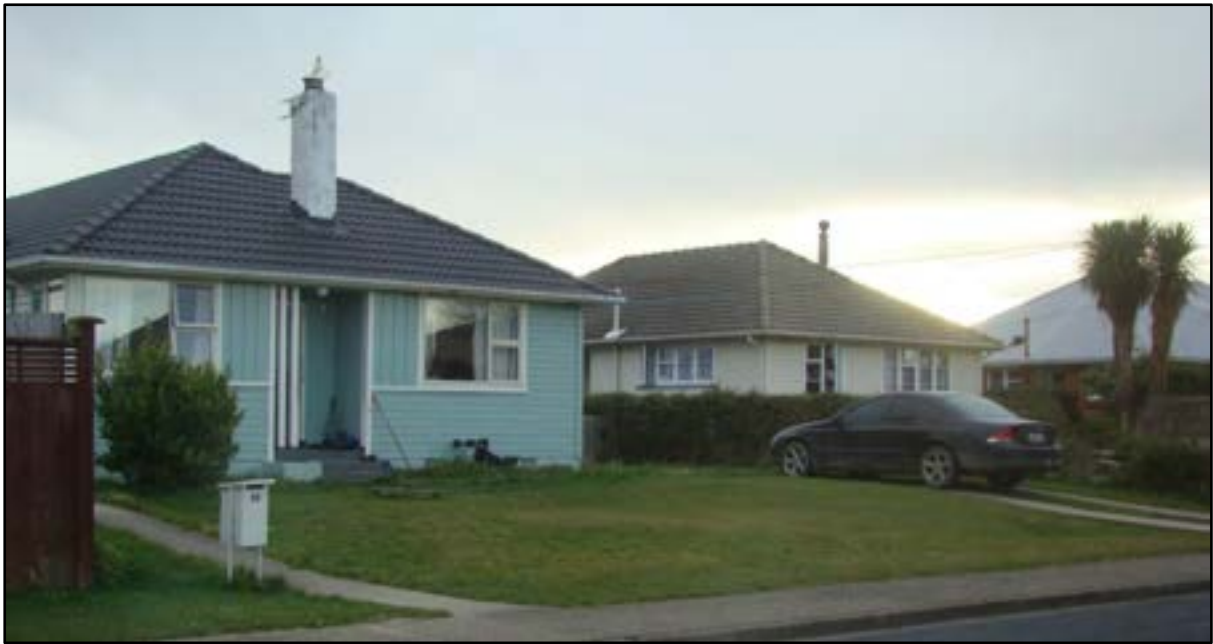
Figure 5: Spey Street (looking south) showing the typical house forms, scale and materials used across the area.
