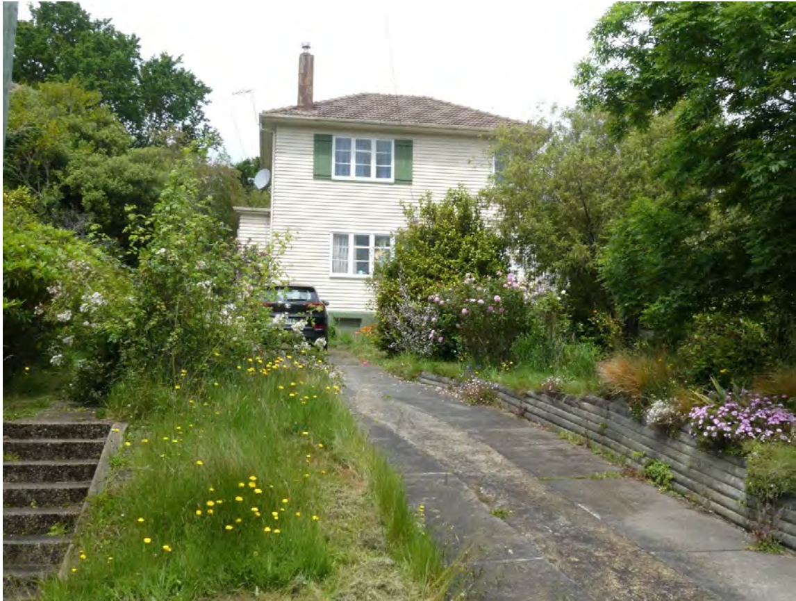
Figure 6: Scarce two-storey house form located on Strathearn Avenue of the same 1938/39 construction period.
