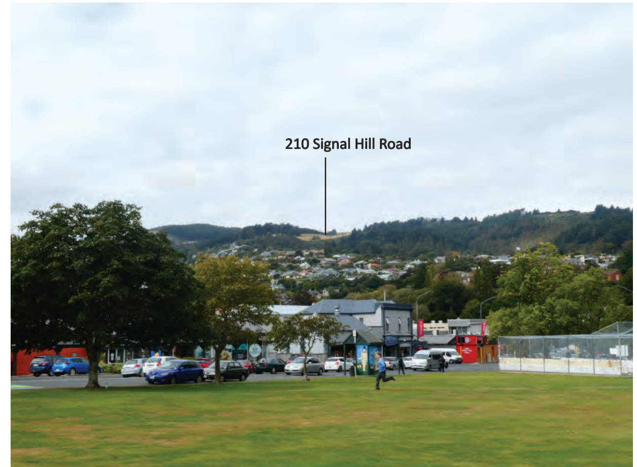
VL 2: View towards site from Gardens Sports Ground.
