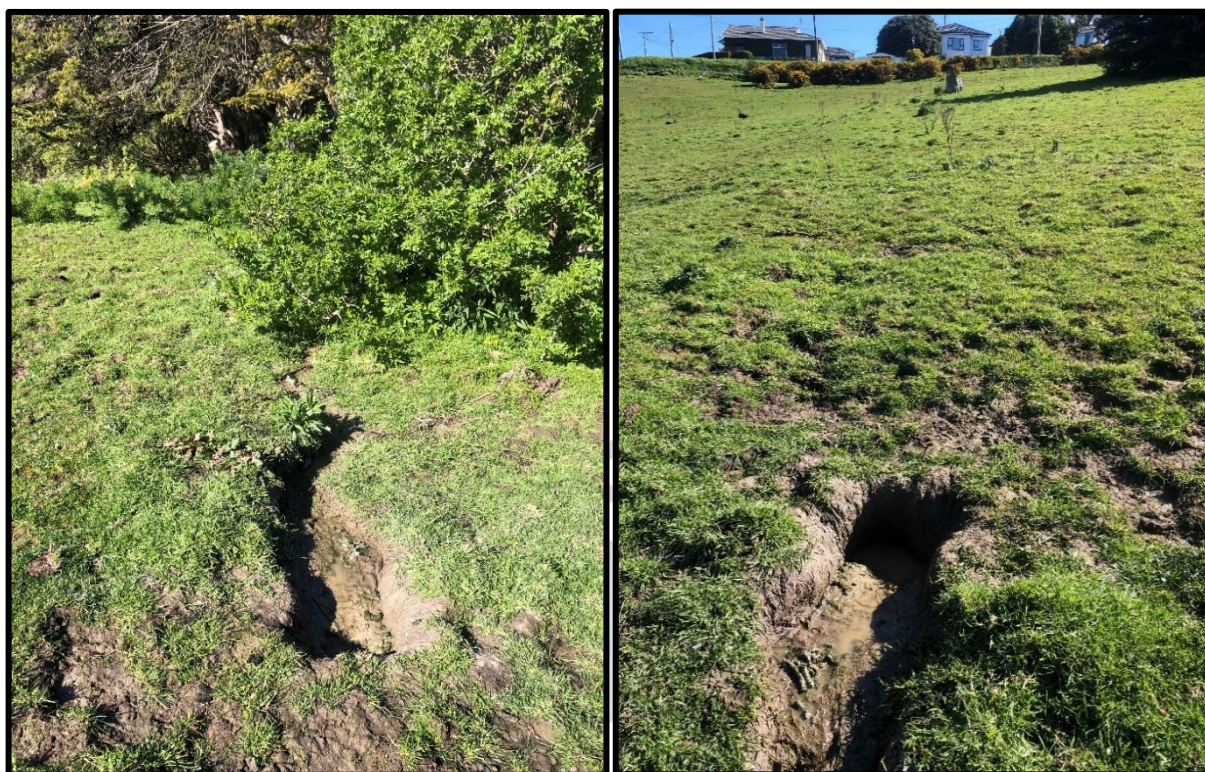
Figure 9: A natural seep approximately 80 m from the Gloucester Street boundary downhill (left) and uphill (right).
