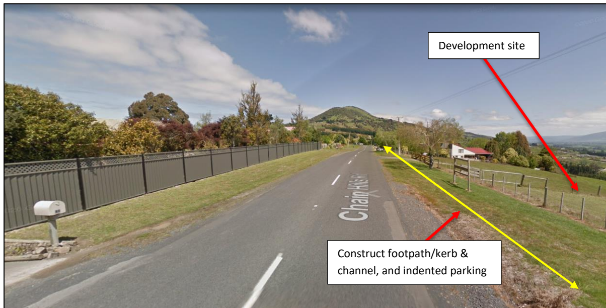
Figure 15 – General scope of proposed footpath to be installed on Chain Hills Road for active road users, adjacent to and opposite the development site. Image looking south-west along Chain Hills Road.
