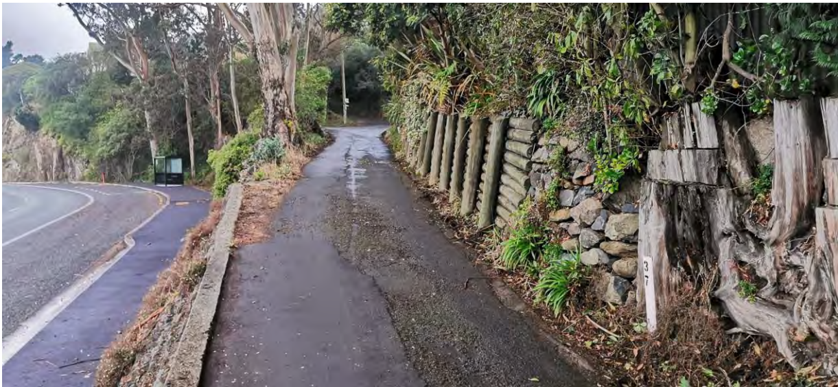
Figure 5 Weller Street existing conditions
