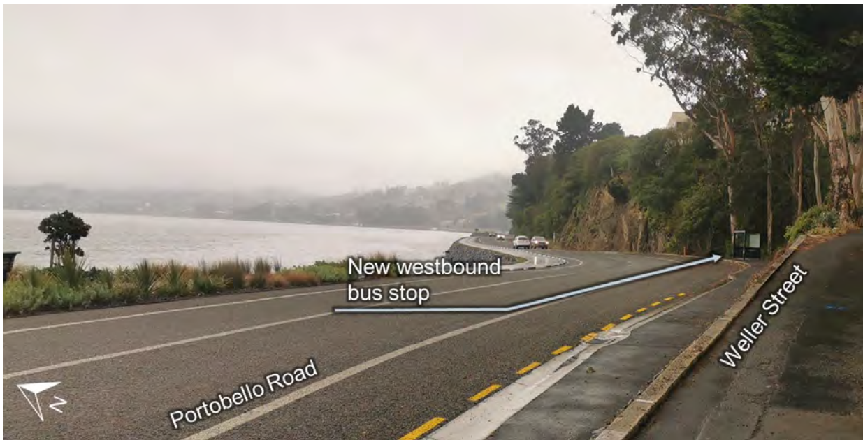
Figure 12 New westbound bus stop located east of Weller Street
