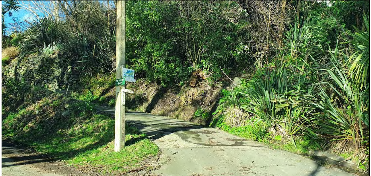
Plate 2: View further up Weller St at single lane accessway to the site with random rubble rock wall in upper area.
