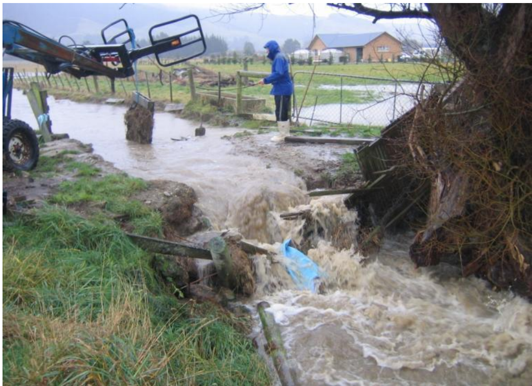
Figure 4. Example of drains and overland flowpaths on the Taieri Plain observed in July 2007. Blockage being removed from a drain
