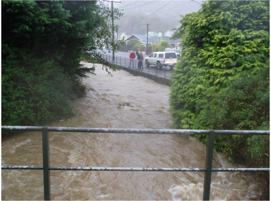
Figure 6. Example of section of channel limited capacity - Lindsay Creek in the vicinity of Palmer Quarry Bridge, looking upstream during a moderate high flow event in July 2017. Flow is less than 20cumecs
