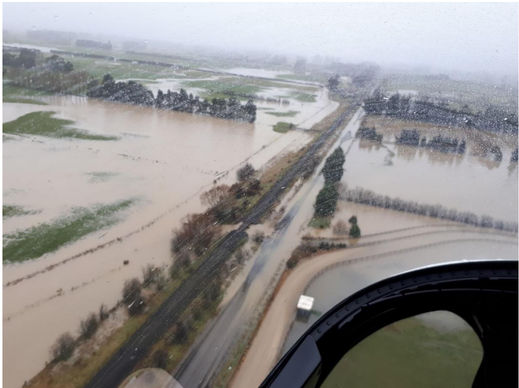
Figure 2. Example of extensive ponding due to Owhiro Stream overtopping its banks and combining with runoff from the hills - Taieri Plain 22 July 2017 – Gladstone Road South and South Island Main Trunk Railway in the foreground. Owhiro Stream in the foreground looking upstream
