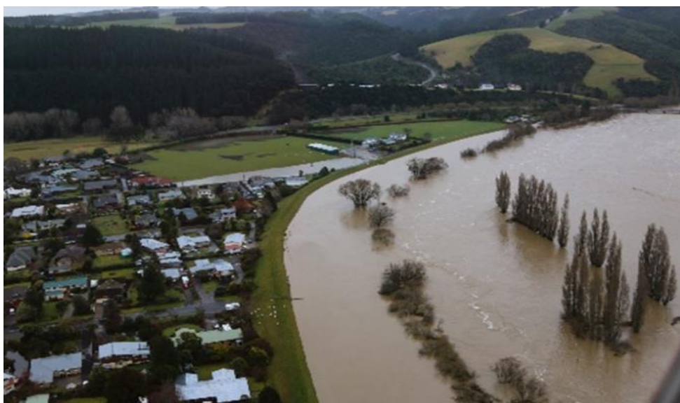
Figure 9: The Lower Taieri Flood Protection Scheme at Outram in July 2017
