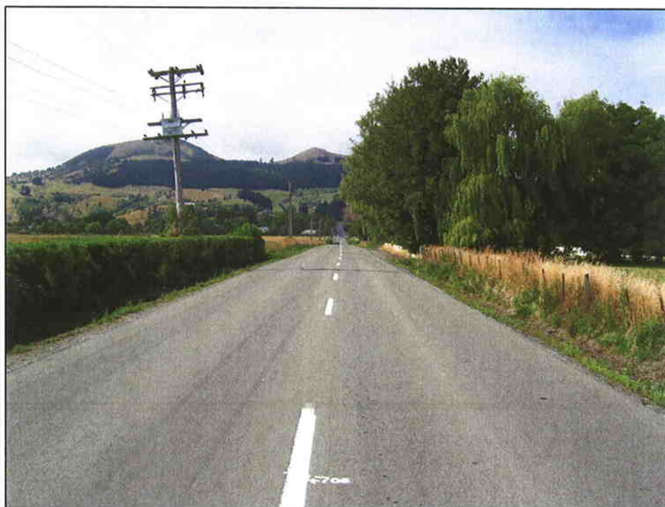
Figure 3-4 : Power poles within clear zone
