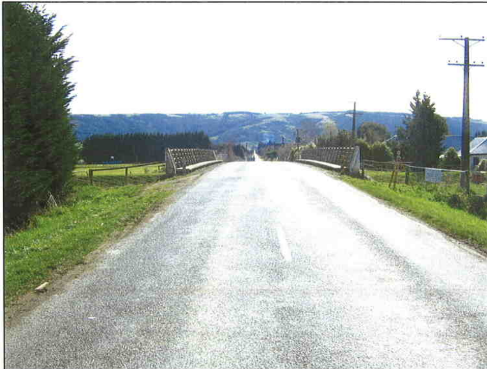
Figure 3-10 : Restricted sight distance at Silver Stream Bridge
