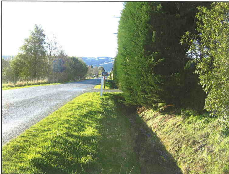
Figure 3-1 : Steep drains within the clear zone
