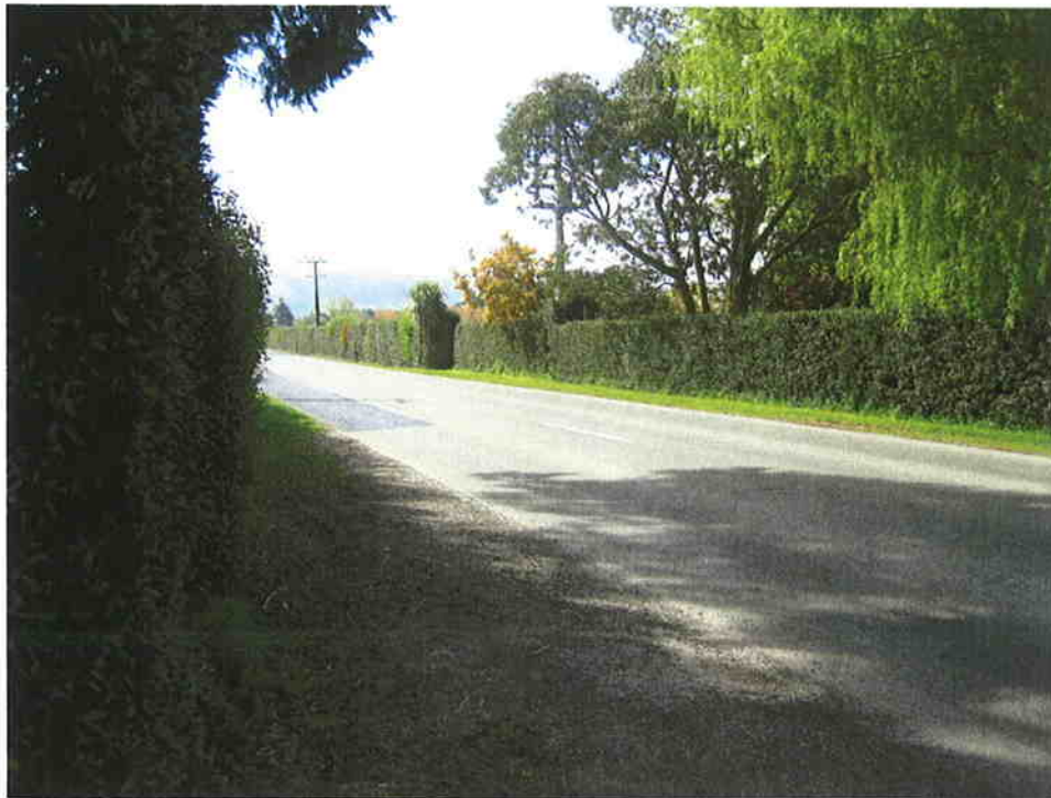
Figure 3-2 : Hedges alongside road limiting sight distance from accessways
