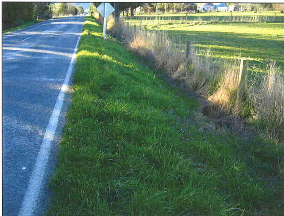
Figure 3-8 : Steep slopes into drains
