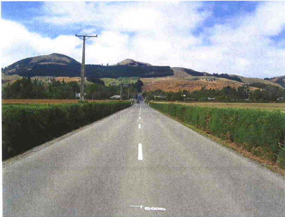
Figure 5-7 : Station 6000. Adjacent to 51 Riccarton Road West Very narrow width between the gorse hedges and service poles close to road. The traffic lanes are narrow and there are no shoulders.
